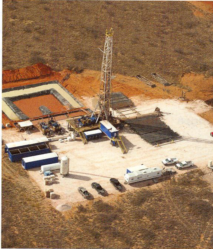
Land Based Drilling Rig
