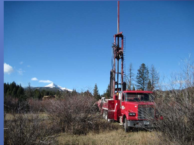
Installation of new monitoring wells
