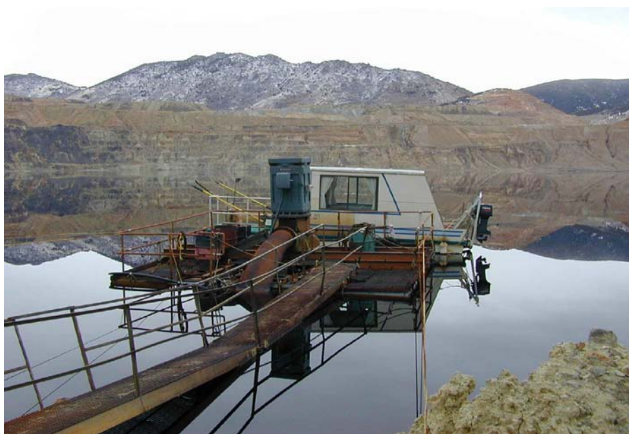
Figure 2-46. MR pontoon boat is used for Berkeley Pit sampling. Boat is docked next to pump station used for pumping pit water to precipitation plant for copper recovery. (Photo courtesy of Daryl Reed, DEQ)
