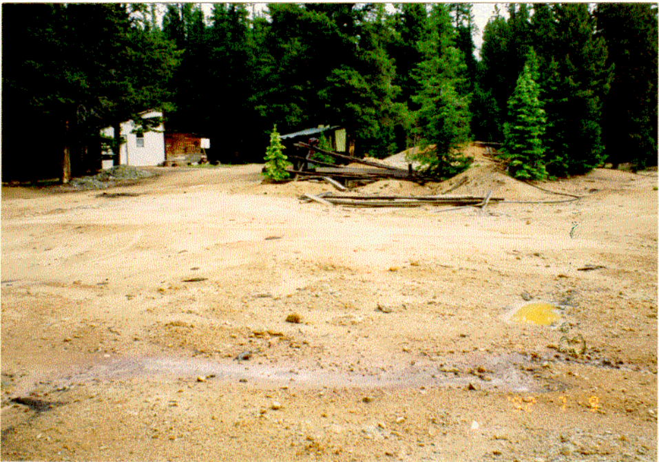
Figure 6A. The west shaft of the North Ada mine is discharging water toward the Cataract Creek drainage; the north shaft was inaccessible. The locations of the photographs are shown in Figure 6.
