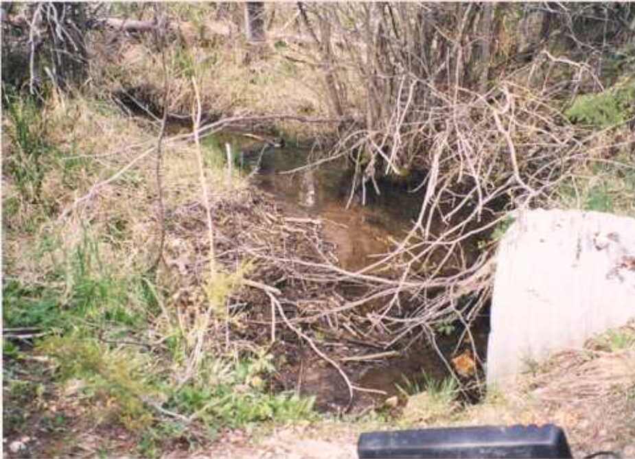
Figure 8b. The lower stretches of Mackay Creek are clear, as sampled (BXXS20M) upstream of the culvert on Forest Road 3323.
