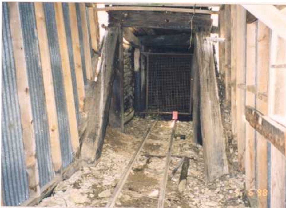
Figure 22c. The adit was open at least for 20 ft and was partially caved beyond that distance, on 05/06/98. The timbers were in good shape.
