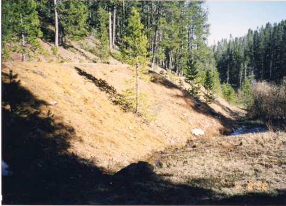
Figure 19a. Mine waste was used in building the road into the Belle of the Castle. The upper reaches of Hensley Creek and the “north fork” of the creek are in contact with the waste.
