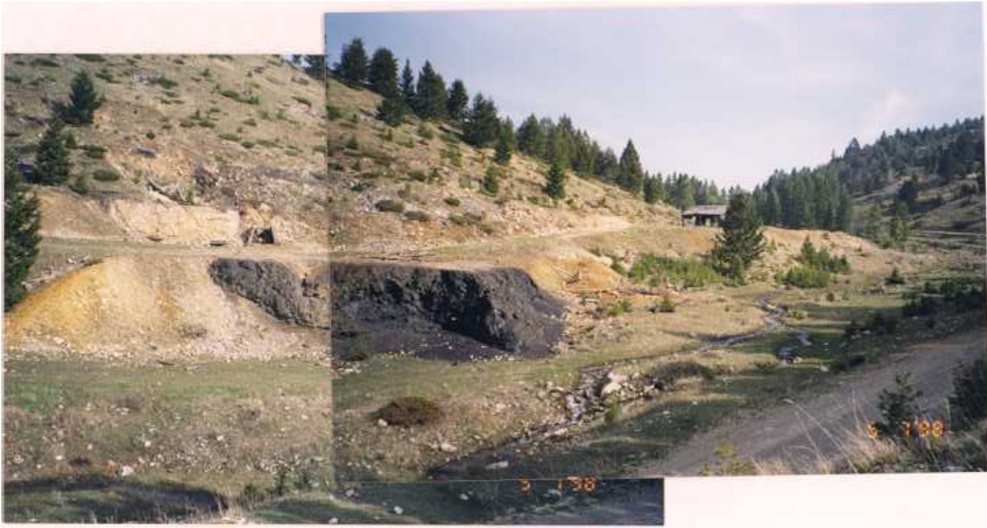
Figure 24a. The black slag on patented land did not directly contact Castle Creek, however, runoff from the slag and waste piles could possibly affect LCNF-administered land. The site is readily visible from Forest Road 581.
