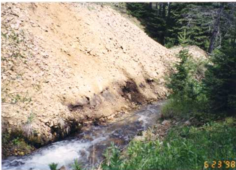
Figure 20a. Hensley Creek eroded the toe of the mine's waste-rock dump when visited 06/23/98. The site was on private land but LCNF-administered land lay both upstream and downstream.
