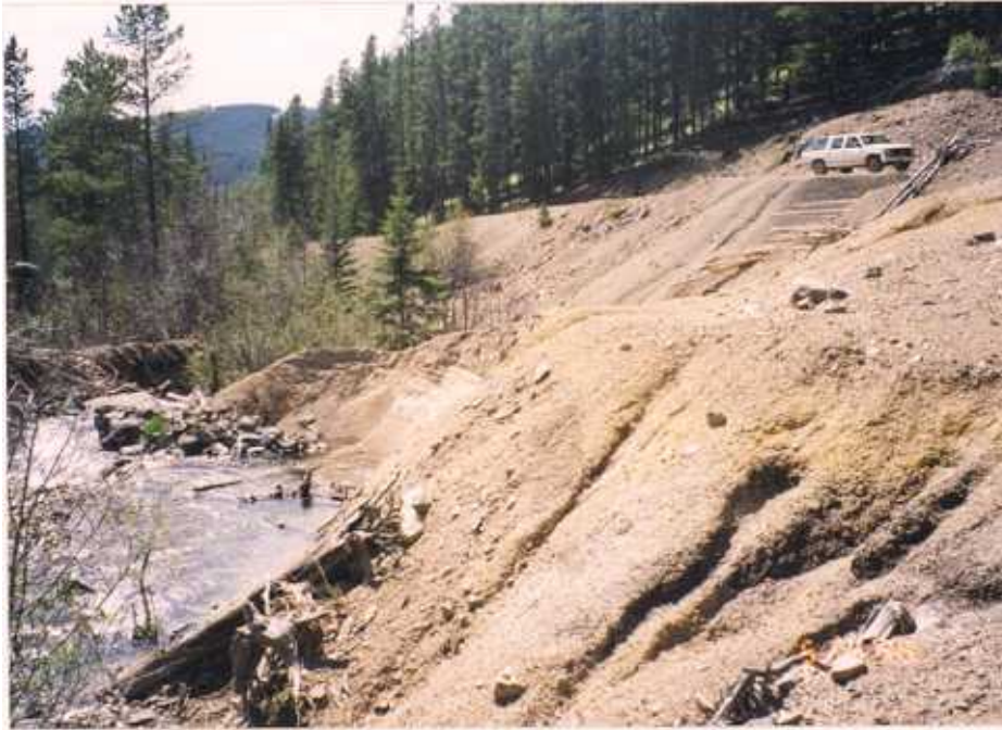
Figure 7a. Carpenter Creek actively erodes the Silver Dyke tailings and runoff has formed rills in the tailings.
