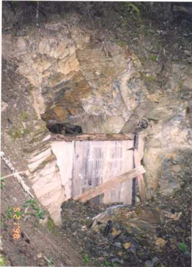
Figure 18a. The adit at Dr. Barnette's Mine had a locked portal but it could be easily circumvented. Rock on the back of the mine had recently spalled off.
