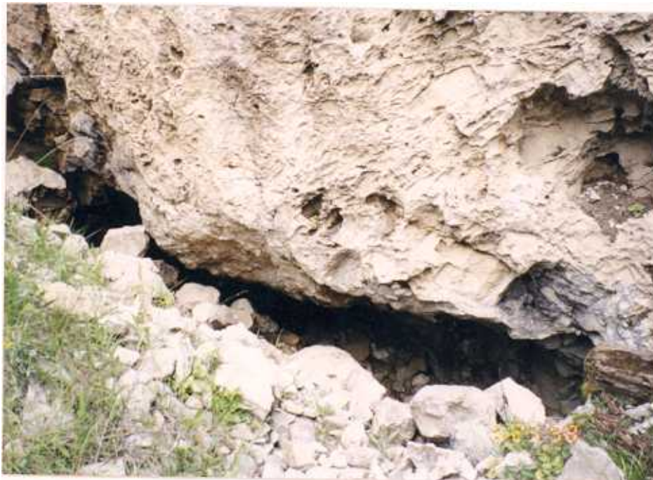
Figure 23b. The portal of the main adit at the Powderly has partially collapsed but an open crawl space still exists.
