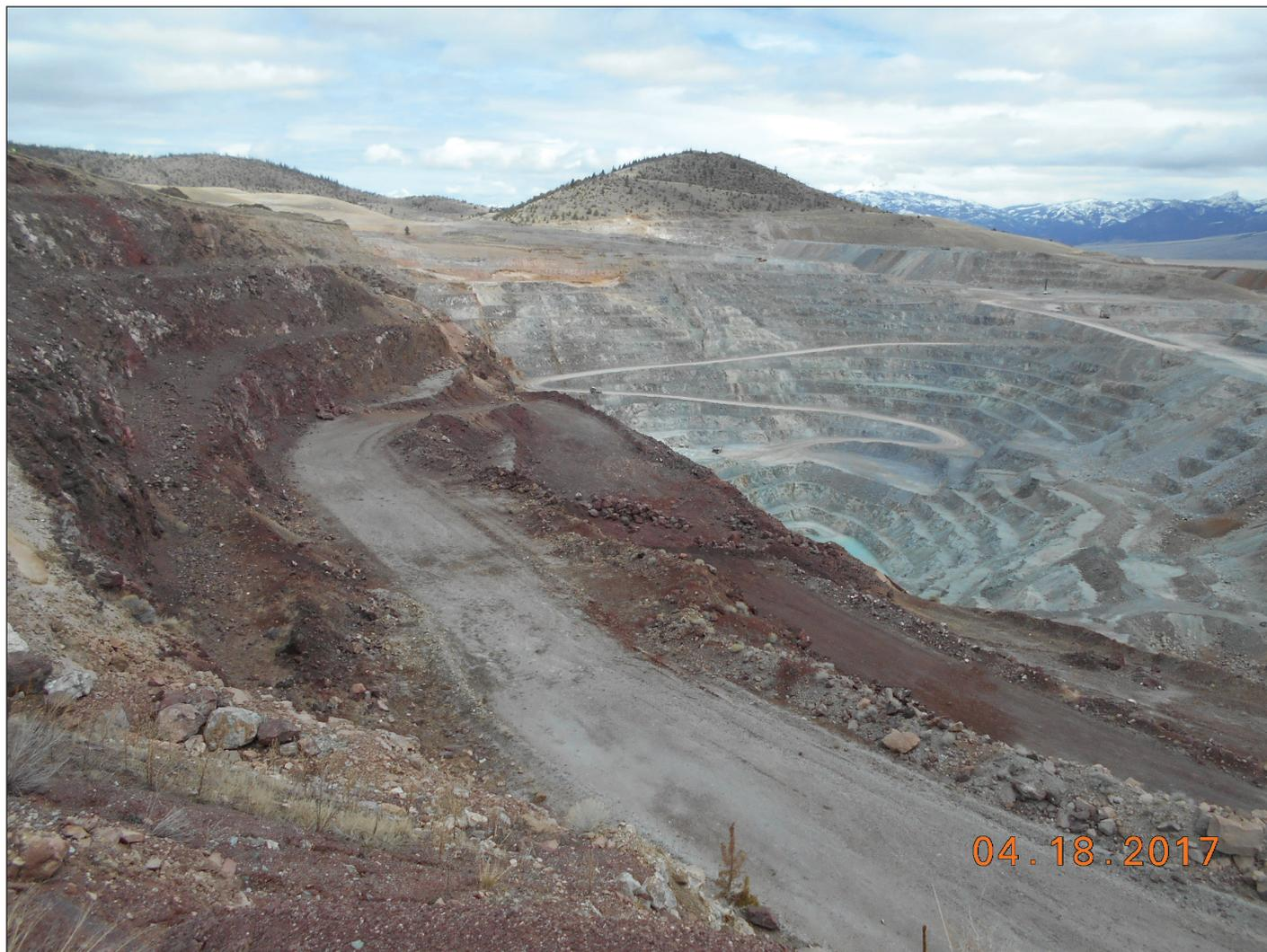
Figure 2. Looking north across the Yellowstone talc mine, operated by Imerys S.A. The Phase 6 pit layback has commenced at the far north end of the pit (upper center of photo), which will expose additional talc ore beneath the upper layers of volcanic tuff and dolomitic waste rock.
