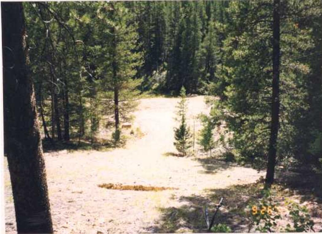
Figure 11a. The Third Term mine has been reclaimed; however, a part of the adit subsided after reclamation (shadow in center of picture).
