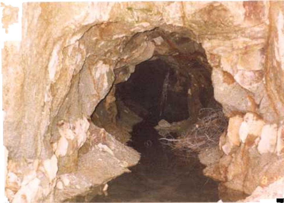
Figure 4a. The adit of the North Ontario mine remained open at least 40 feet from the surface. The tunnel was partially flooded and discharged water on to the dump.
