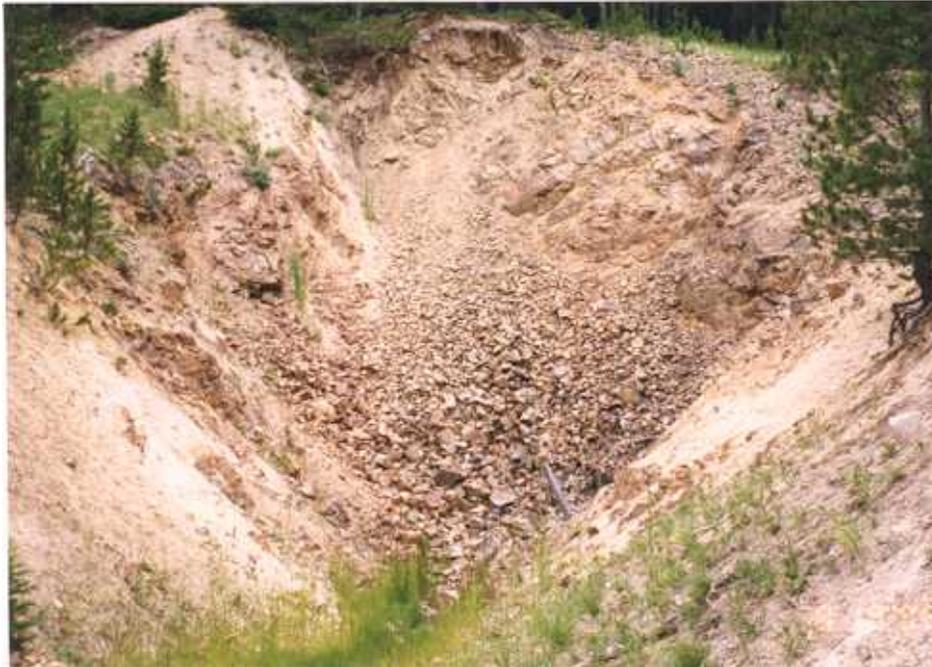
Figure 7a. The collapsed adit at the Hope mine discharged about 1 gpm. The highwall was steep but generally stable.
