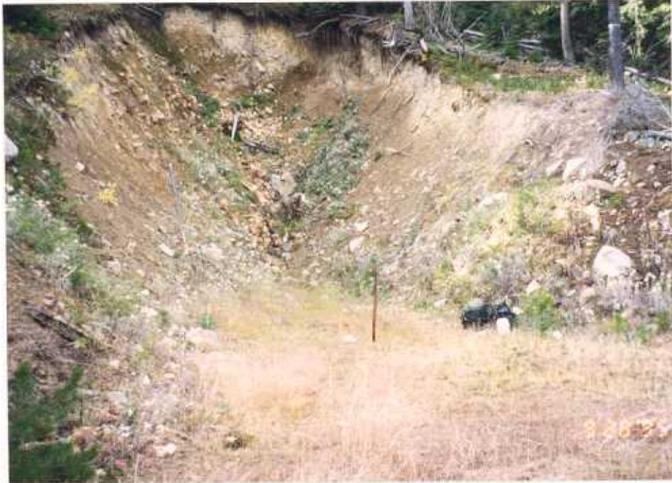
**Figure 10a.** The collapsed adit of the Viking mine discharged about 0.5 gpm. No other discharges were observed on or near the site.
