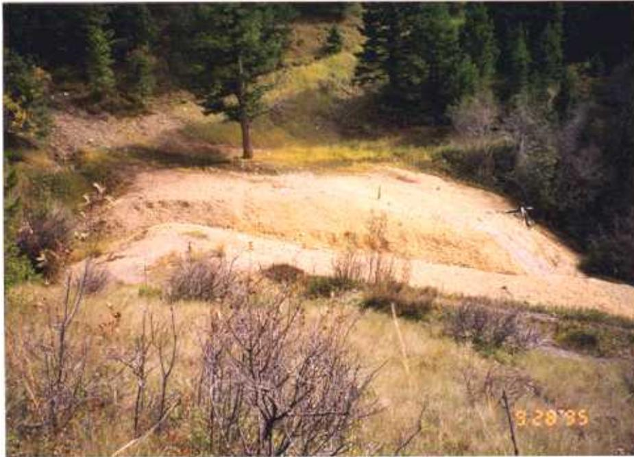
Figure 30a. A channel cut through the waste of the Mammoth mine; an adit discharge/seep appears in the upper left of photo and flows to the right at the edge of the waste dump.
