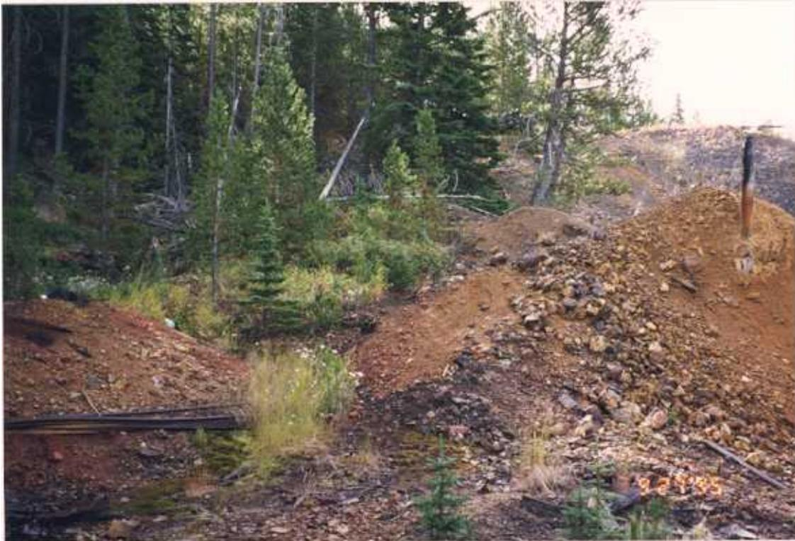
Figure 13a. The lower, caved adit of the Monarch mine was discharging a small amount of water on to the lower waste-rock dump. The adit lies in the trees just left of center.
