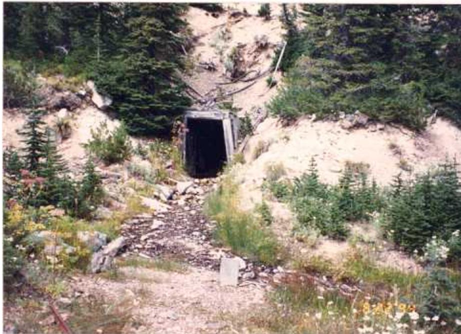
Figure 29b. Five-gpm discharge emerged from the lower Copper Camp adit that was caved beyond the lagging.
