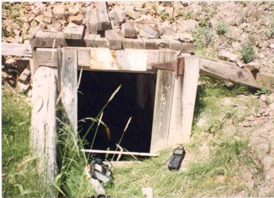
Figure 24a. Water stands in the open, timbered, and lagged adit at the Bobby Boy with a  $<0.5$ -gpm discharge.
