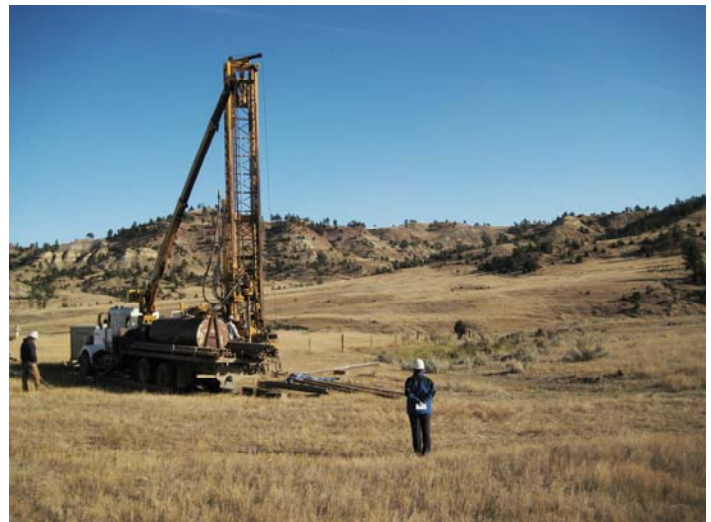
Drilling monitoring wells in southeastern Montana.
