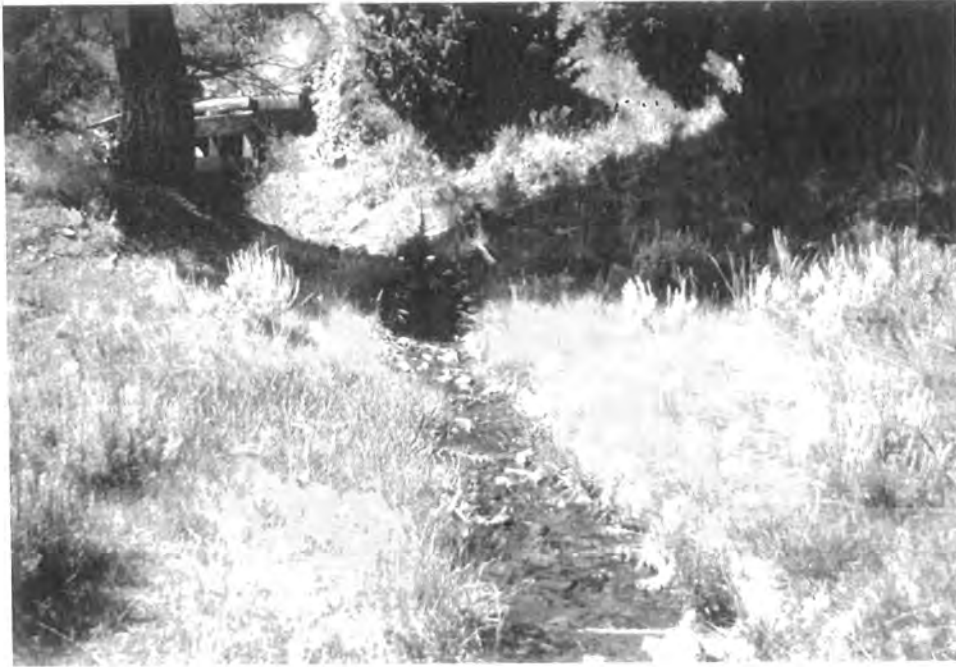
Figure 9.10 A large discharge flows from the partially collapsed adit at the Iron Mask mine and mill.
