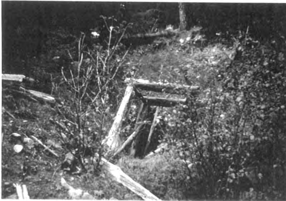
Figure 5.9 A small, intermittent discharge flows from the collapsed upper adit at the Redwing site.
