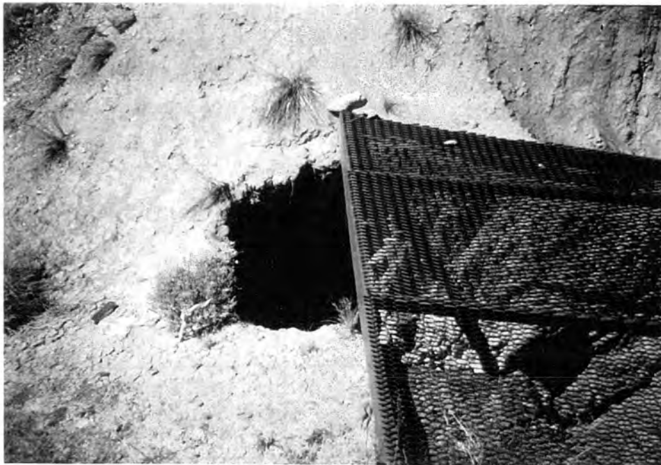
Figure 2.7 An open shaft immediately south of the main tailings impoundment has been sealed with a steel grate; however, caving of soil and rock around the edges of the grate have made the shaft hazardous once again.
