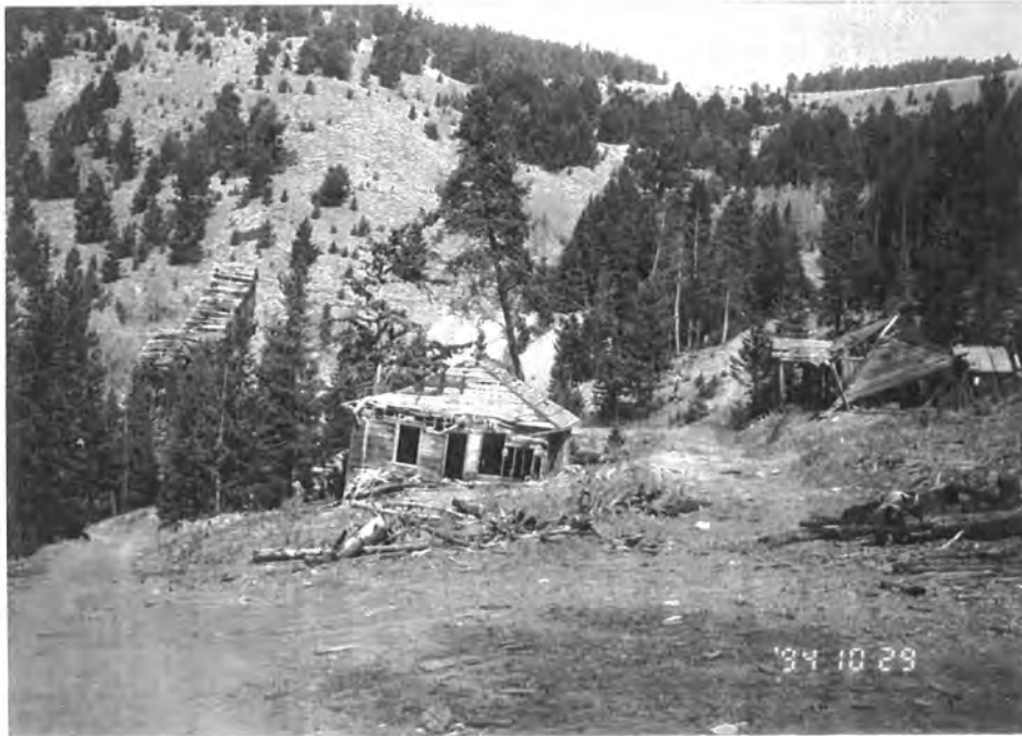
Figure 10.5 Delapidated mine buildings and a waste-rock dump at the Marrietta mine.
