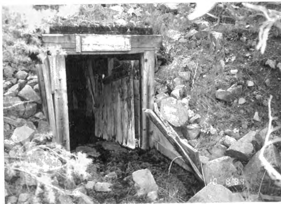
Figure 4.9 A discharge flows from the open portal at the Charcoal (Shawbut) mine.
