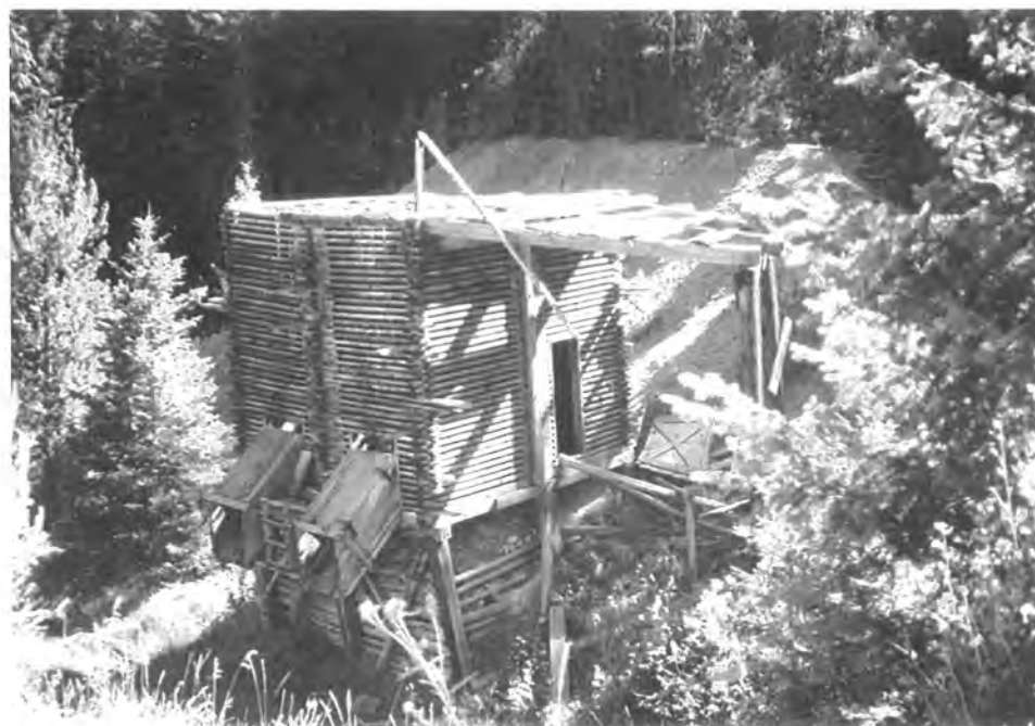
Figure 10.3 An ore bin at the Bartlett mine next to a waste-rock dump. Note the vegetation growing on top and at the bottom edge of the dump.
