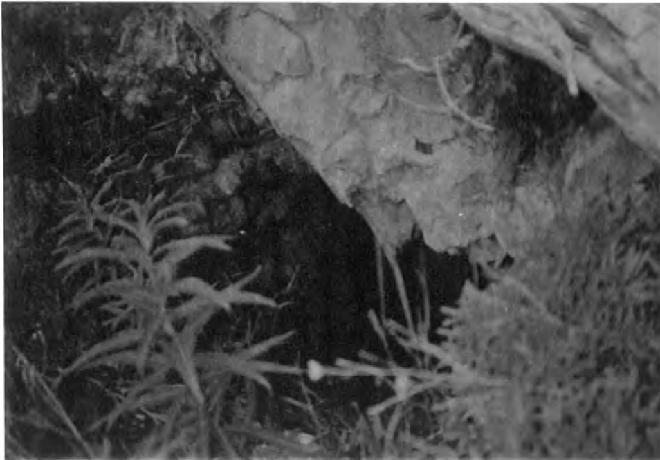
Figure 6.20 The open adit at the Unnamed 12N14W11DABB mine has a small discharge that flows across the top of the waste-rock dump.
