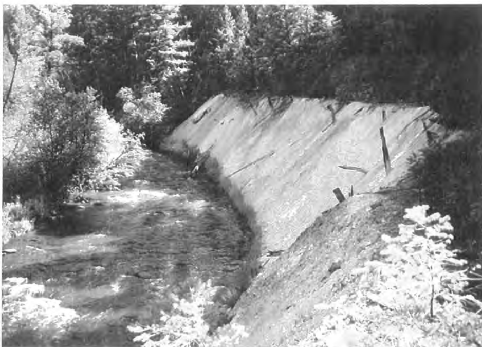
Figure 6.10 Flint Creek is actively eroding the streamside waste-rock dump at the Londonderry mine and mill.
