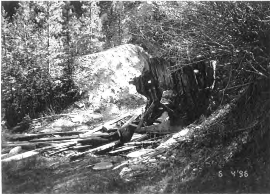
Figure 9.12 A discharge flows from the collapsed adit at the Ottawa mine.
