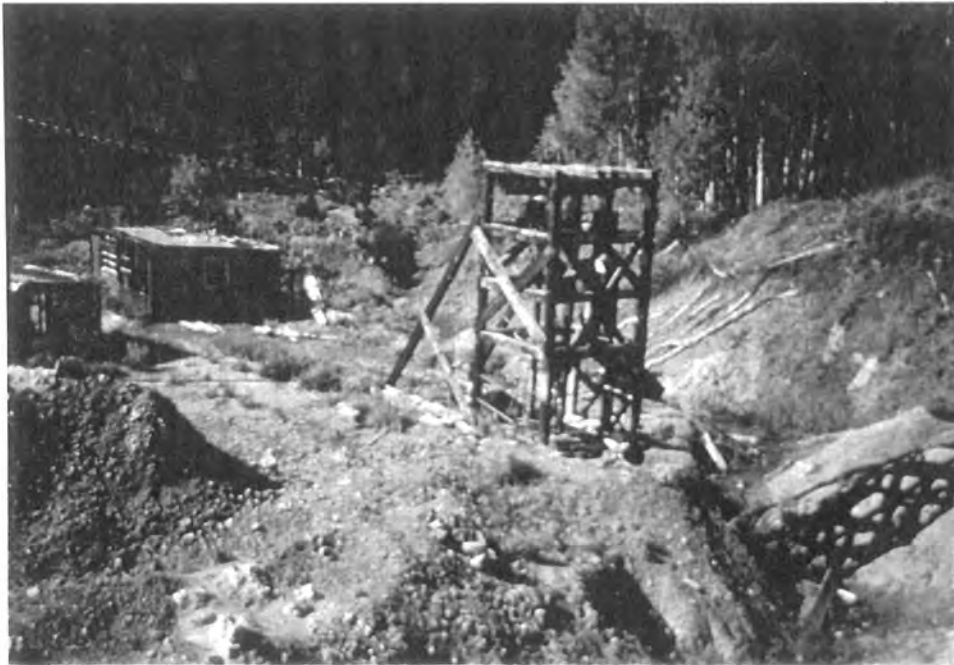
Figure 5.23 A seep begins near the flooded shaft and flows into a marshy area southeast of the mine.
