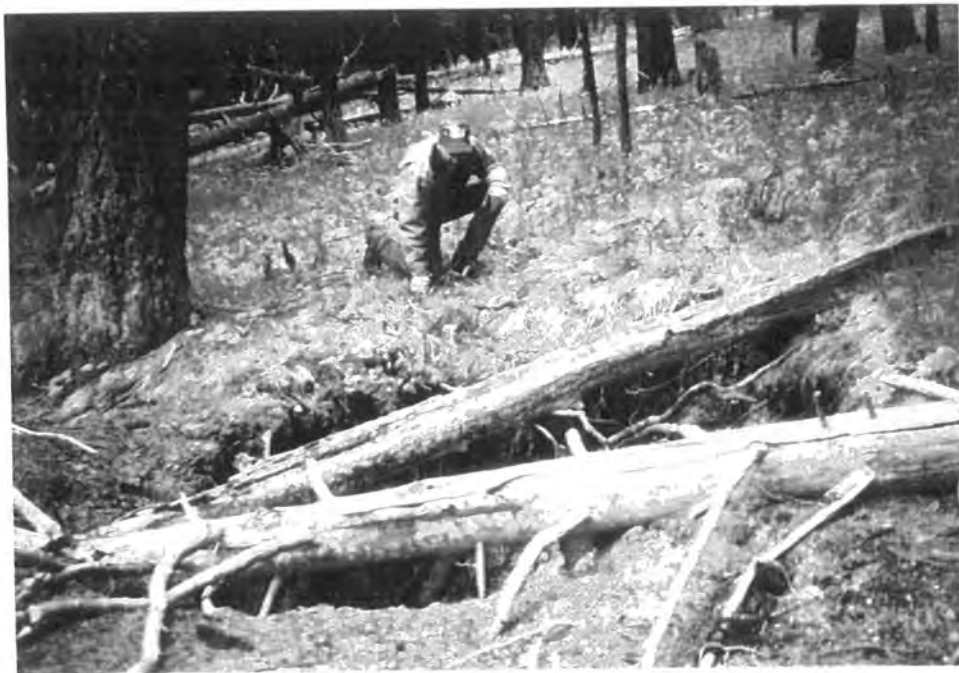
Figure 4.4 Several hazardous mine openings are located around the site, including this collapse feature associated with adit A4.
