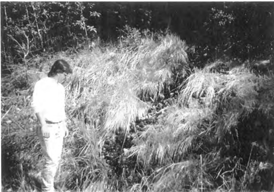
Figure 6.16 The discharge from the A3 adit flows down the embankment next to the road. No vegetation is growing within the discharge channel.
