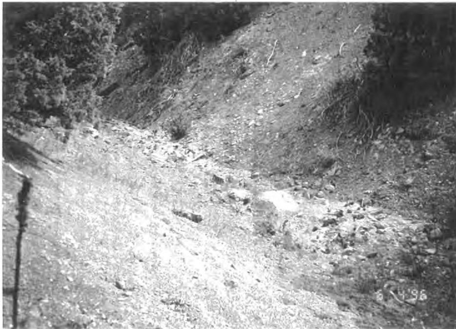
Figure 9.3 A small, milky seep surfaces along the ephemeral drainage just below the lowermost waste-rock dump.
