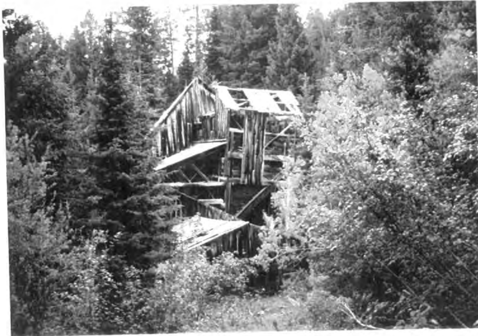
Figure 4.3 The mill building at the Mountain View is in poor condition.
