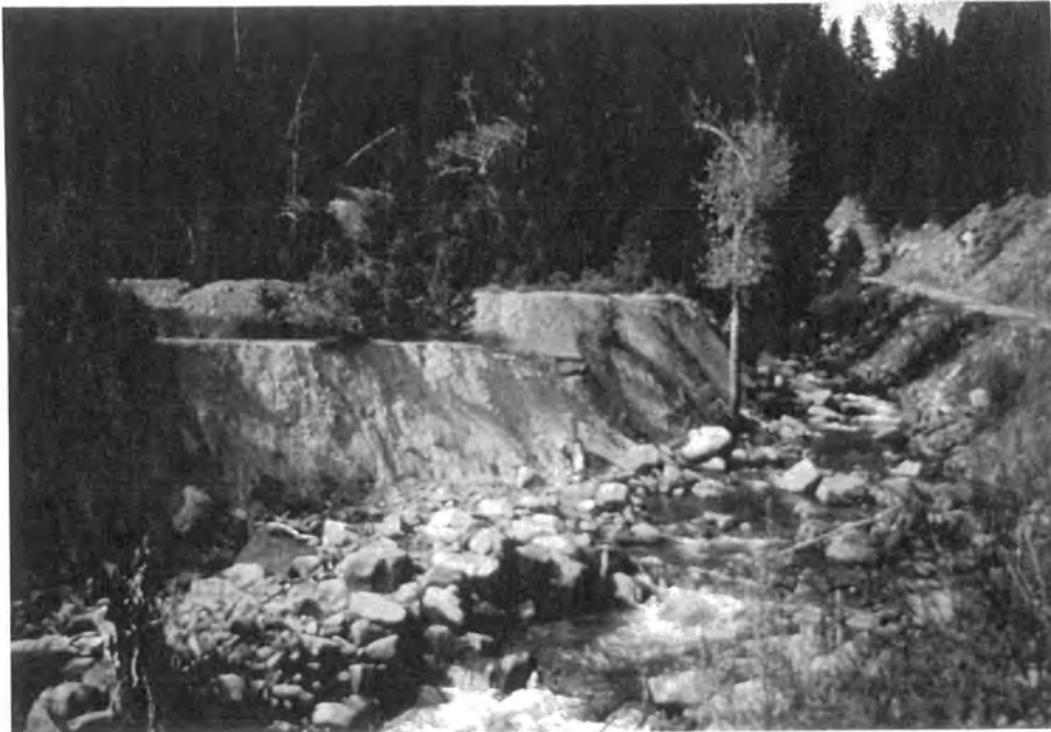
Figure 5.15 A large streamside waste-rock dump is being actively eroded by Cataract Creek at the Mantle mine.
