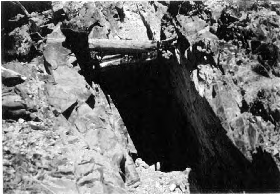
Figure 3.19 A pool of water is located in an open stope at the Hidden Treasure mine.
