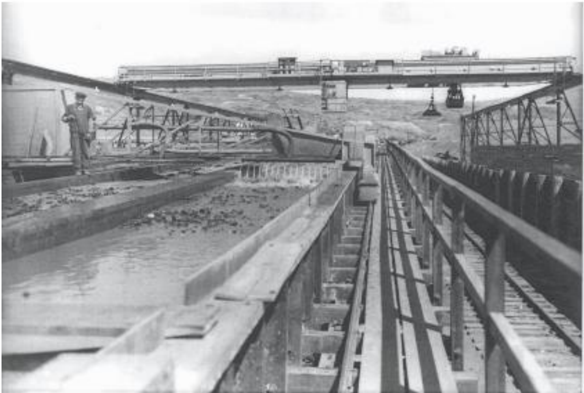
Figure 1-6. Precipitation plant scrap iron in contact with underground mine discharge water. (Photo courtesy World Museum of Mining, Butte, Montana.)
