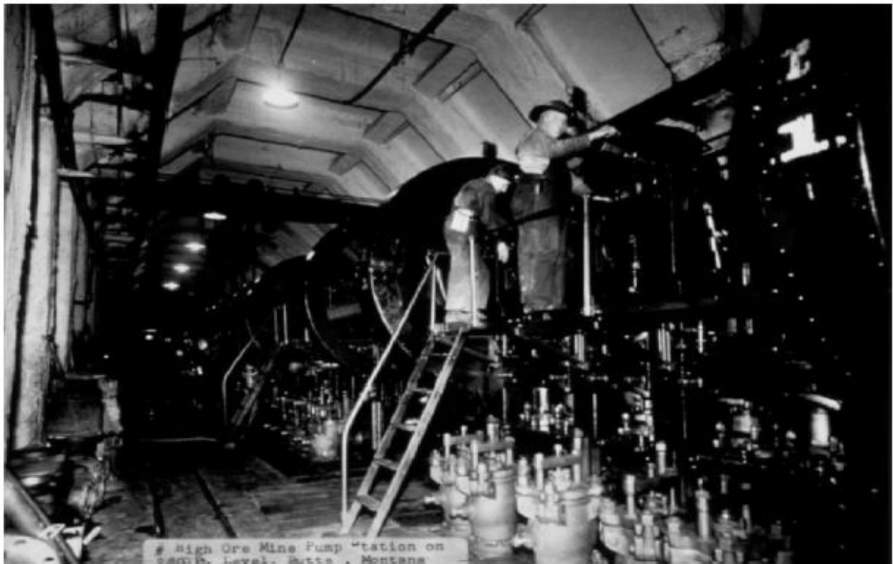
Figure 1-1. High Ore Mine pump station, 2,800-ft level. (Photo courtesy World Museum of Mining, Butte, Montana.)
