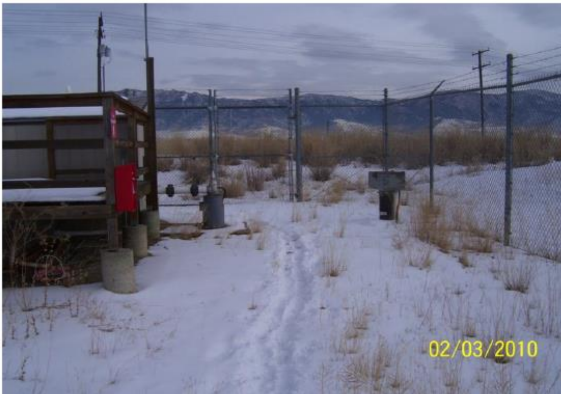
Figure 4-2. West Camp pump station 1997–2011.
