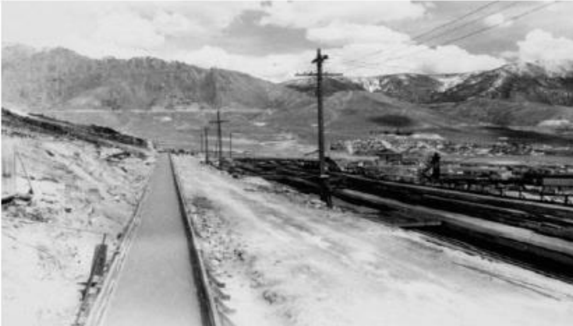
Figure 1-5. Flume conveying water pumped from Butte underground mines to precipitation plant. (Photo courtesy World Museum of Mining, Butte, Montana.)
