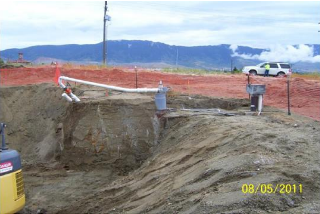
Figure 4-3. West Camp pumping well, discharge line, and monitoring well exposed during 2011 construction activities.
