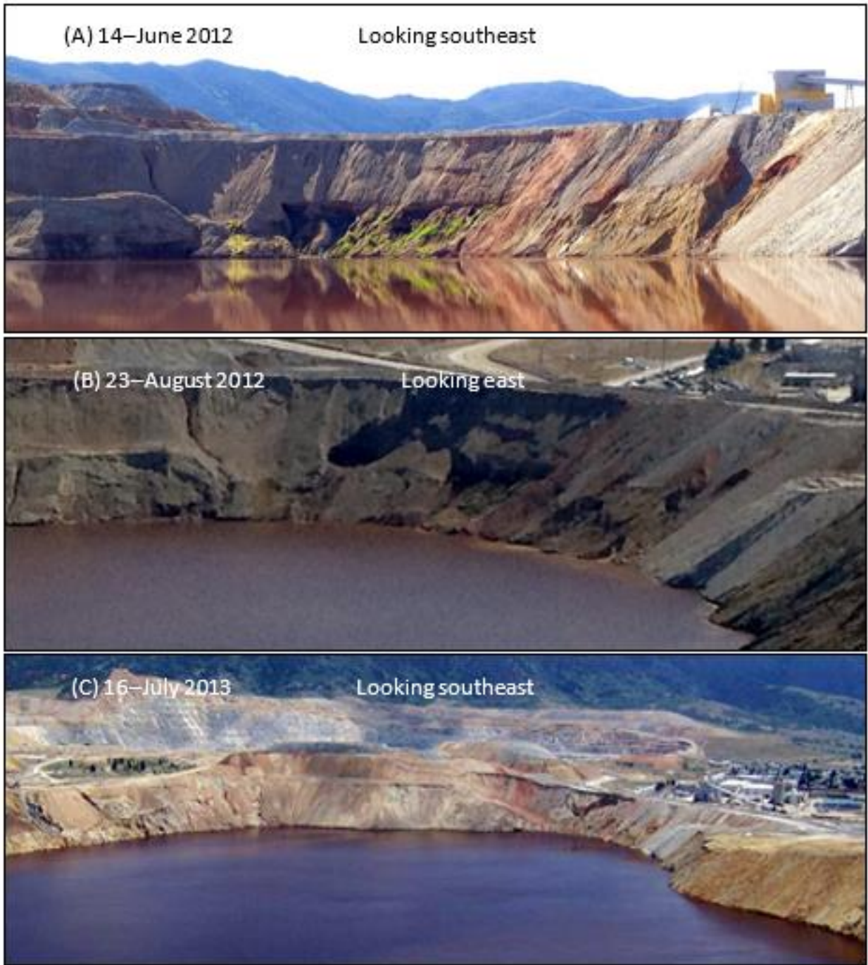
Figure 3-25. Pictures of the southeast corner of the Berkeley Pit prior to the 2012 landslides (A) and after the August 2012 (B) and February 2013 (C) events.
