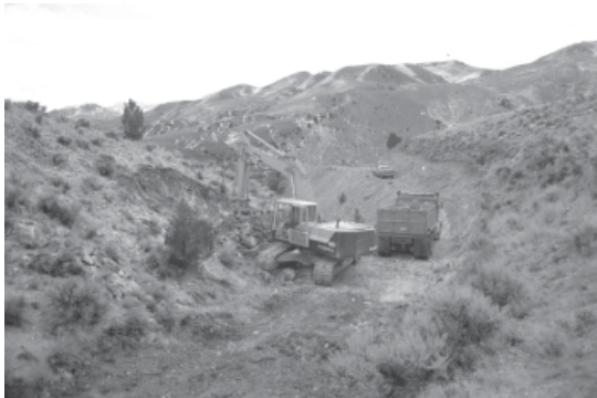
Figure 37. Excavation of bulk sample from the 134 deposit, Grasshopper Creek.
