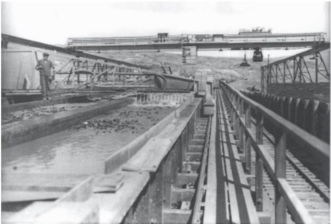
Figure 1-6. Precipitation plant scrap iron in contact with underground mine discharge water.
