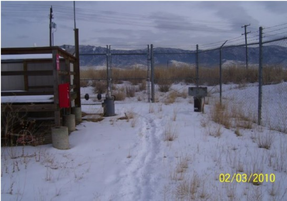
Figure 4-2. West Camp pump station 1997–2011.
