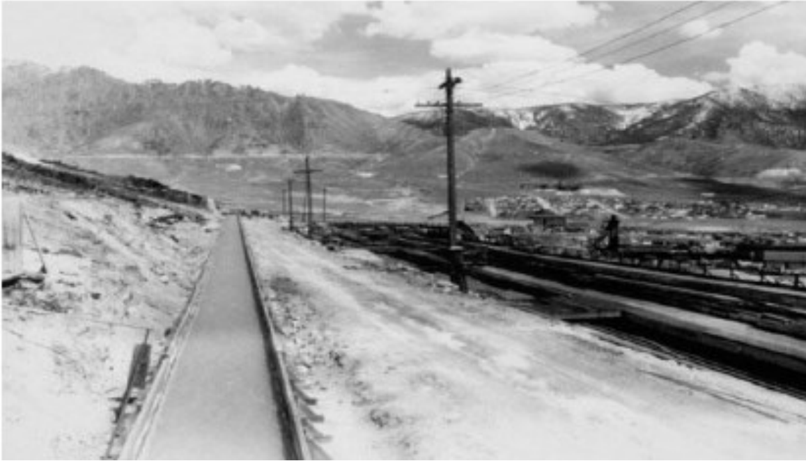
Figure 1-5. Flume conveying water pumped from Butte underground mines to precipitation plant.
