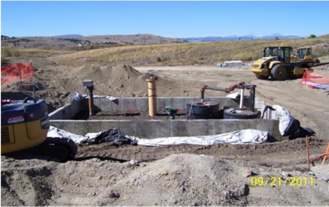
Figure 4-4. West Camp construction activities showing a new pump station foundation and infrastructure improvements surrounding the pumping well and discharge line.
