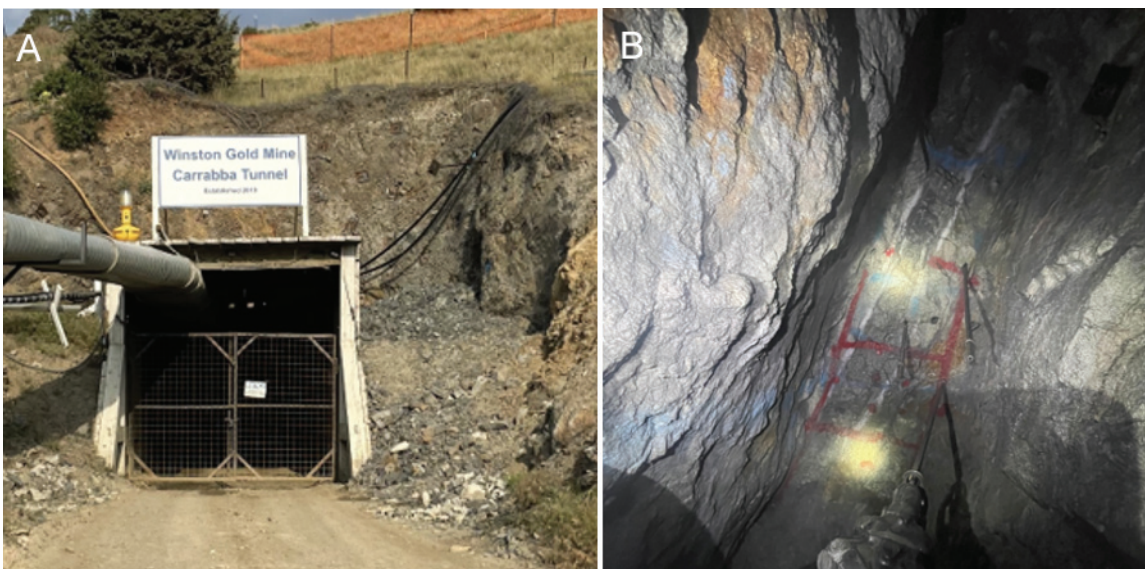
Figure 3. Photographs of the most recent mining operations, including the new Carrabba Tunnel (left) and an underground view of a narrow, steeply dipping sulfide vein (right).
