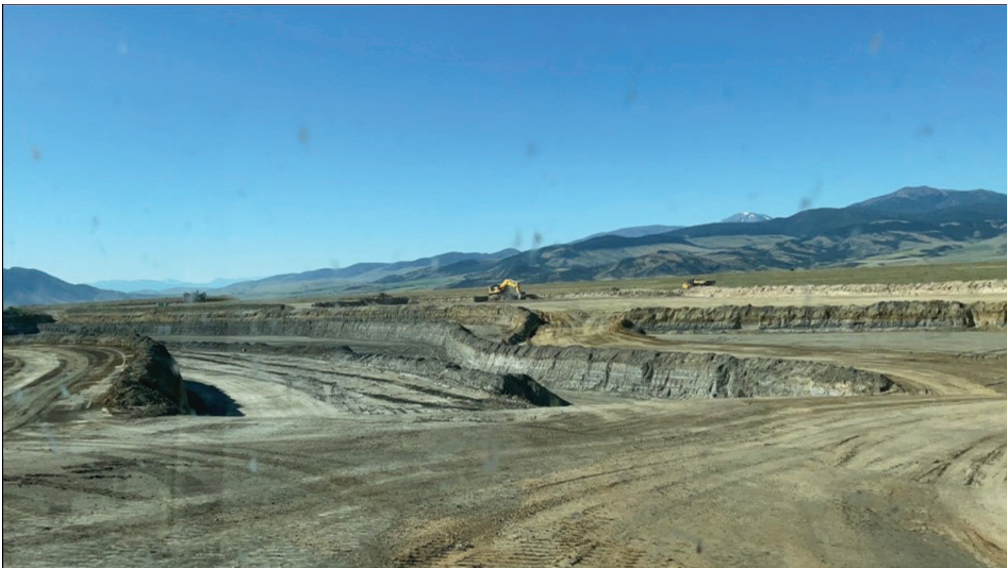
Figure 3. Excavation of the tailings from TSF-1 at the Golden Sunlight Mine. The existing reclamation soil cap being salvaged for future use, following the removal and reprocessing of waste from the unlined facility.
