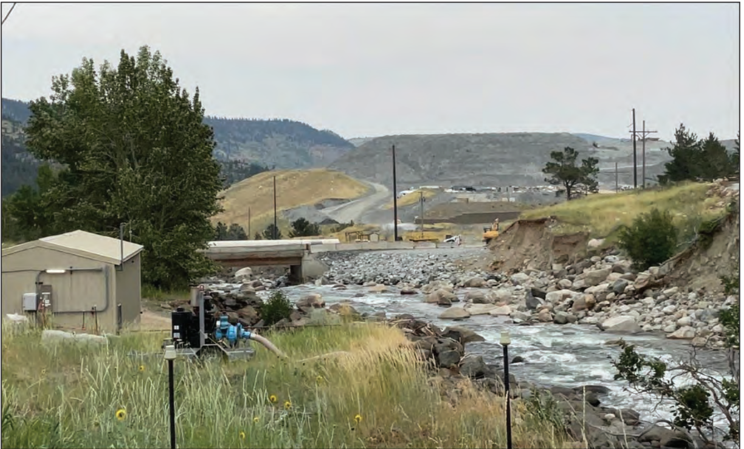
Figure 4. From August 2022 site inspection, the bridge repair at the Stillwater Mine nearing completion following the June flood.
