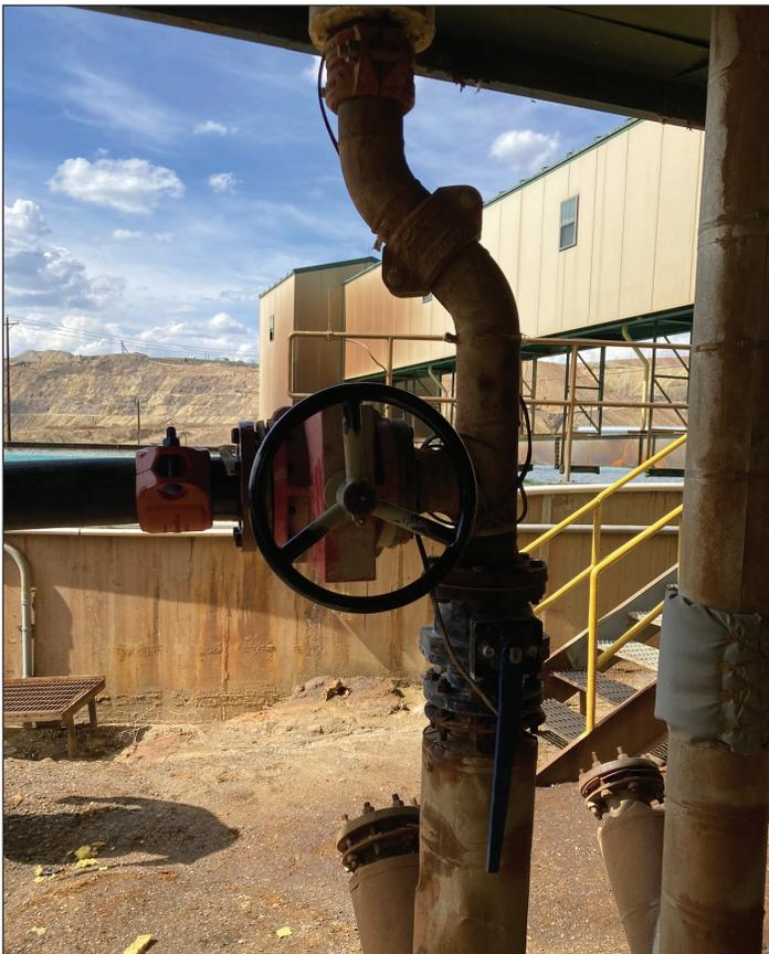
Figure 5. Modification to the Stage Two discharge line for transport of solids to geotubes.
