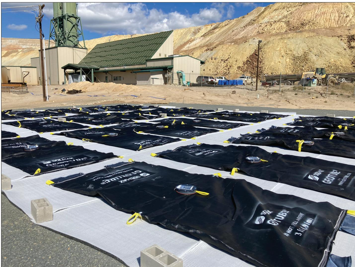
Figure 10. Geotubes arranged in a 4 x 6 grid with HsB WTP and manifold in background.
