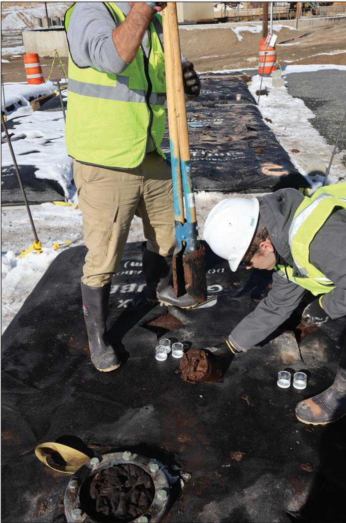
Figure 23. Removing core of HPC using post hole digger (Bird, in process, with permission).
