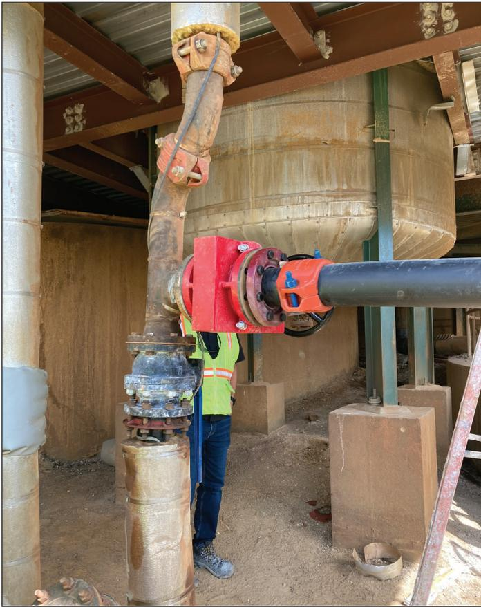
Figure 3. Modification to the Stage Two discharge line for transport of solids to geotubes.
