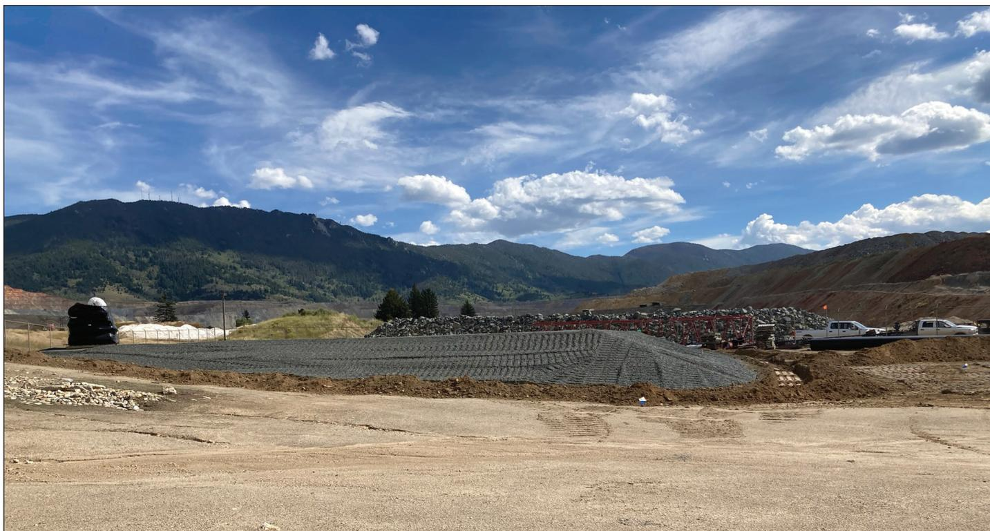
Figure 6. Gravel pad at HsB used as geotube laydown area.
