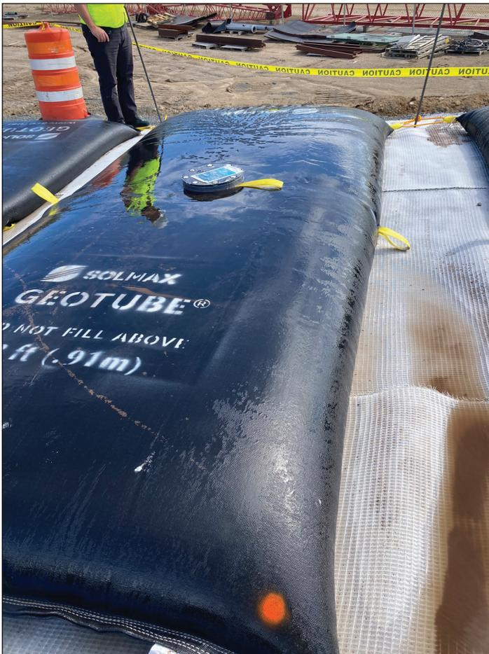
Figure 17. Geotube filled to capacity and dewatering sludge, 09/25/2023.
