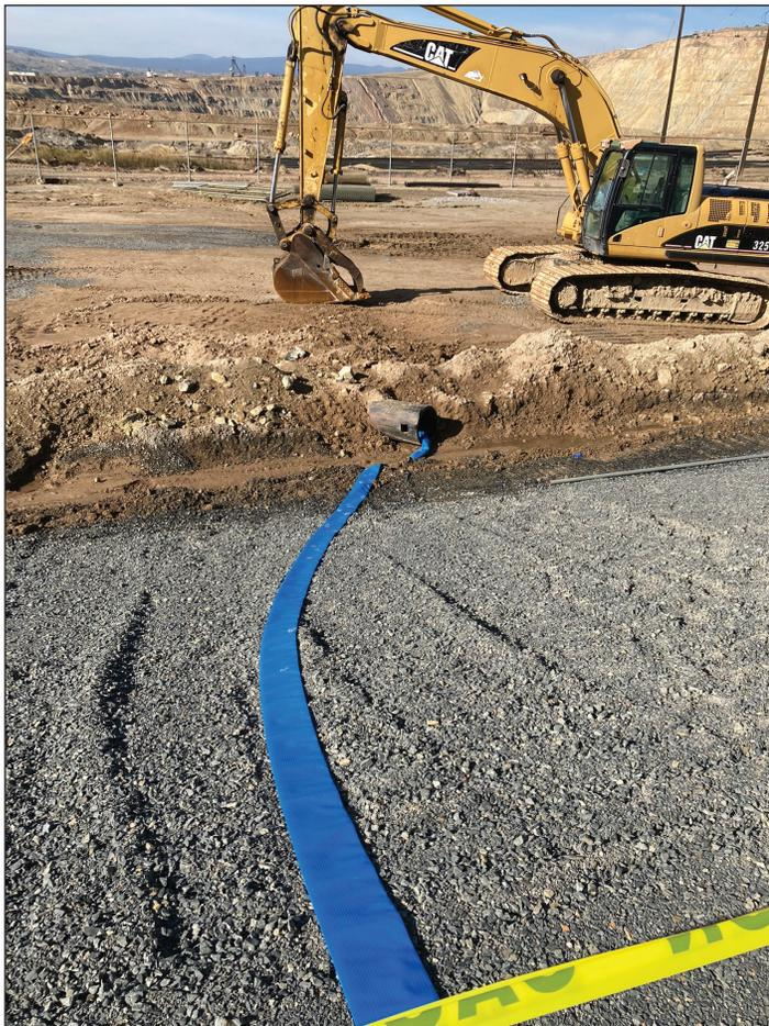
Figure 9. Drainage pipe located in western ditch of gravel pad.
