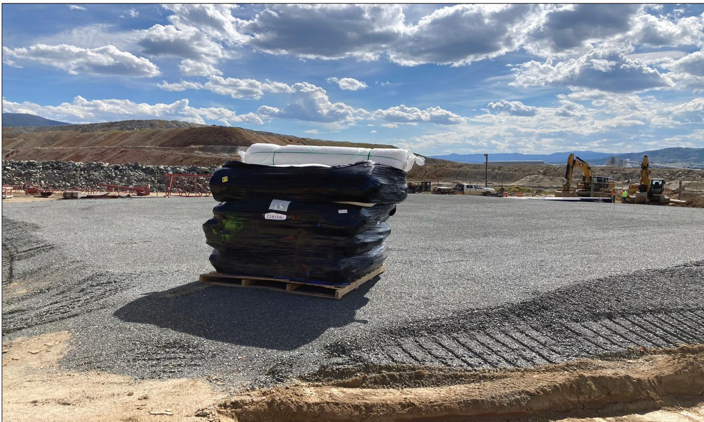
Figure 7. Gravel pad with packaged geotubes in forefront.
