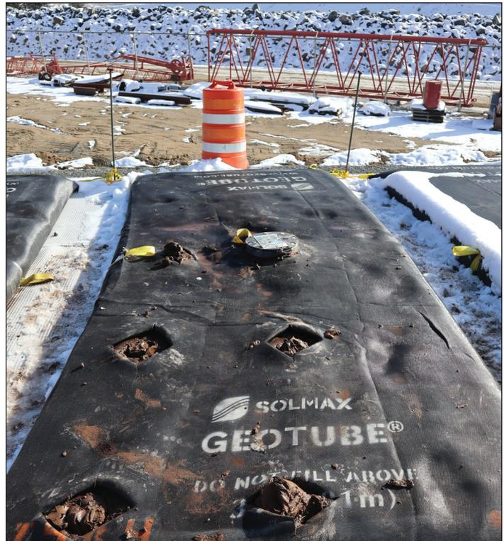
Figure 26. Geotube after sampling event (Bird, in process, with permission).
