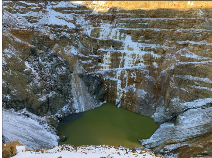
Figure 3-9. The pit at the Golden Sunlight Mine.
