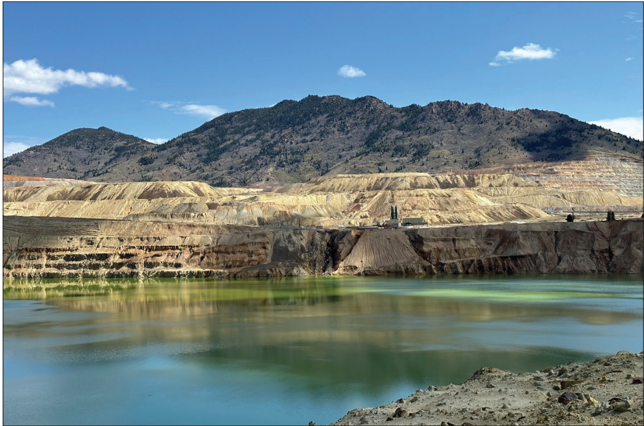
Figure 3-1. The Berkeley Pit and the Horseshoe Bend Water Treatment plant.
