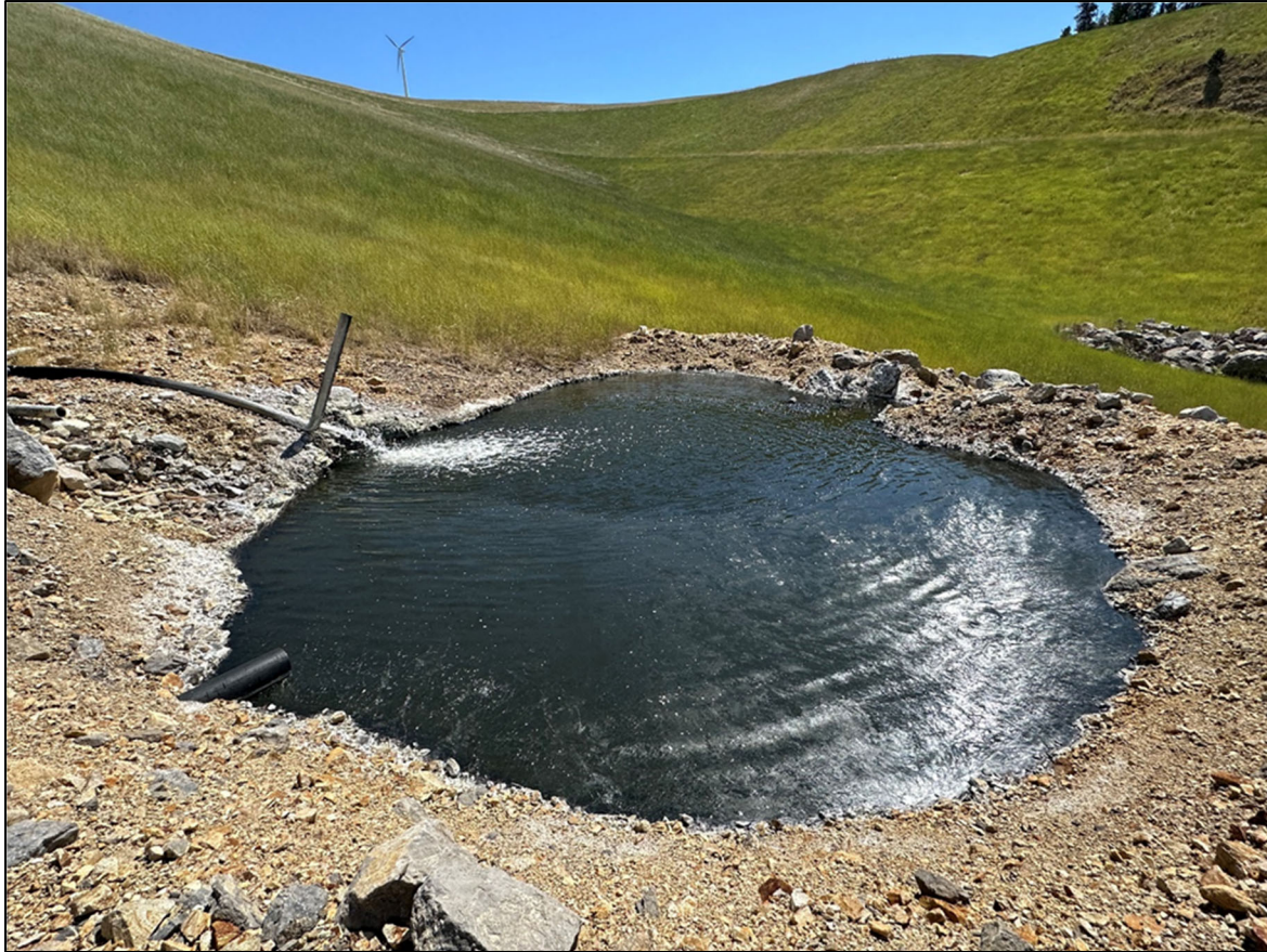
Figure 4. Zortman-Landusky water treatment plant discharge, Phillips County.
