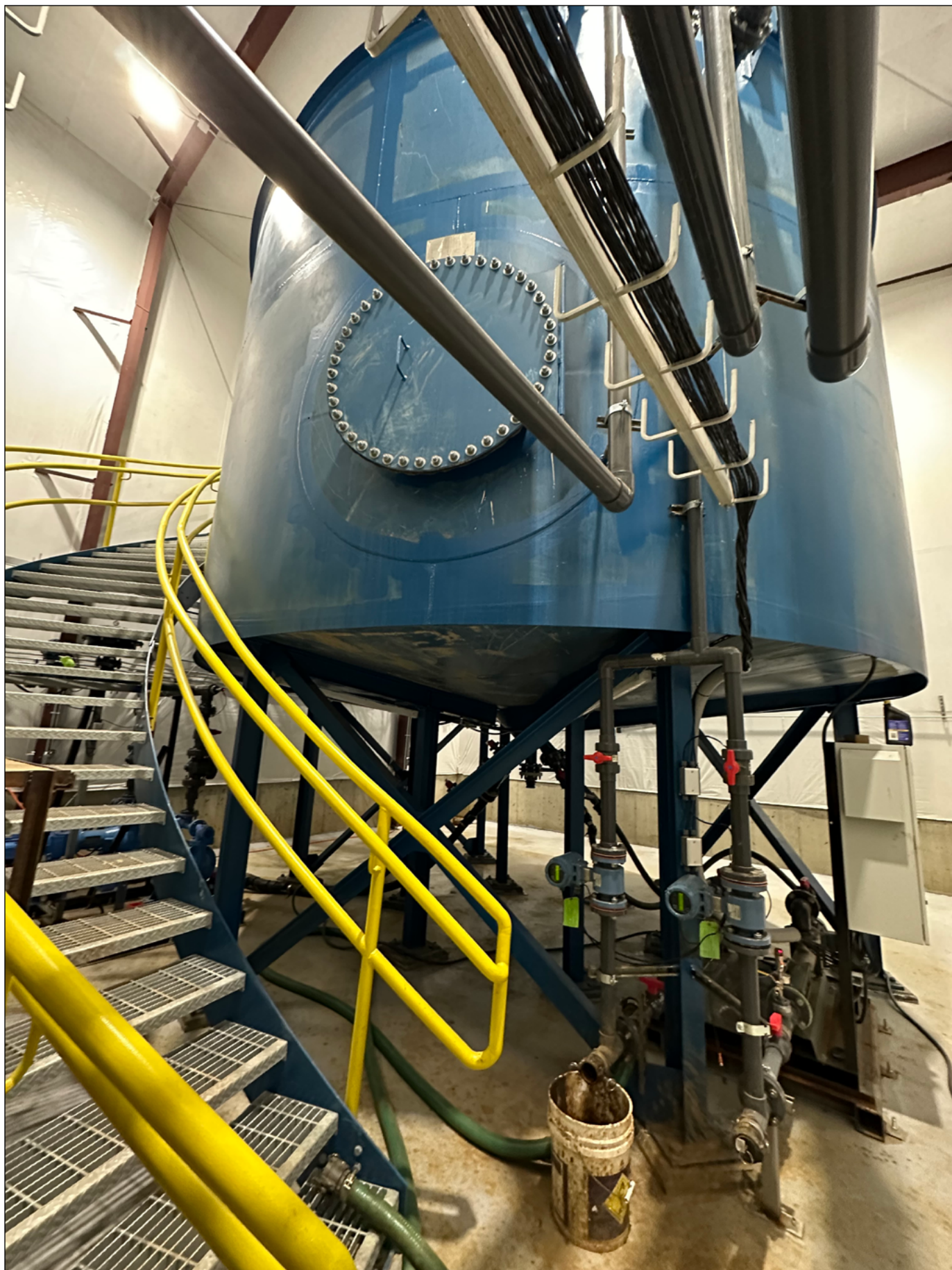
Figure 3-23. Mike Horse Mine: clarifier inside the Mike Horse Mine water treatment plant.
