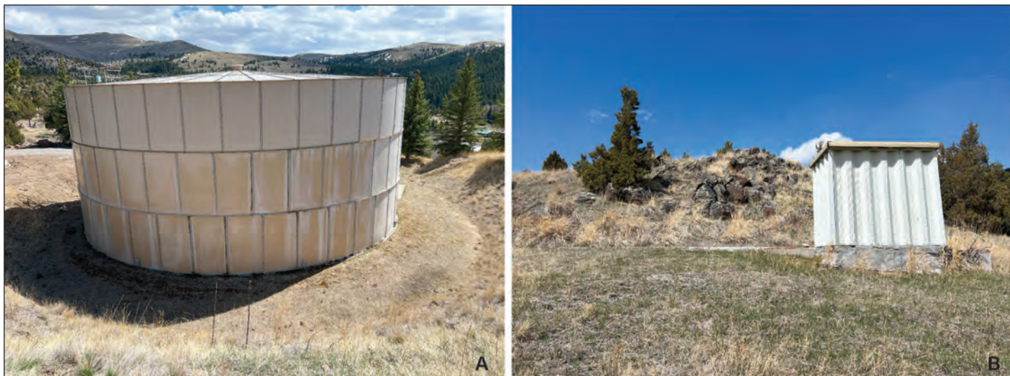
Figure 9. Water infrastructure at STOP 5. (A) The main water tank for the town. Water is treated before entering this tank. When it is full, water is diverted into an overflow channel. (B) The pump house, located at the contact between lava flows (uphill) and tuff (downhill).
