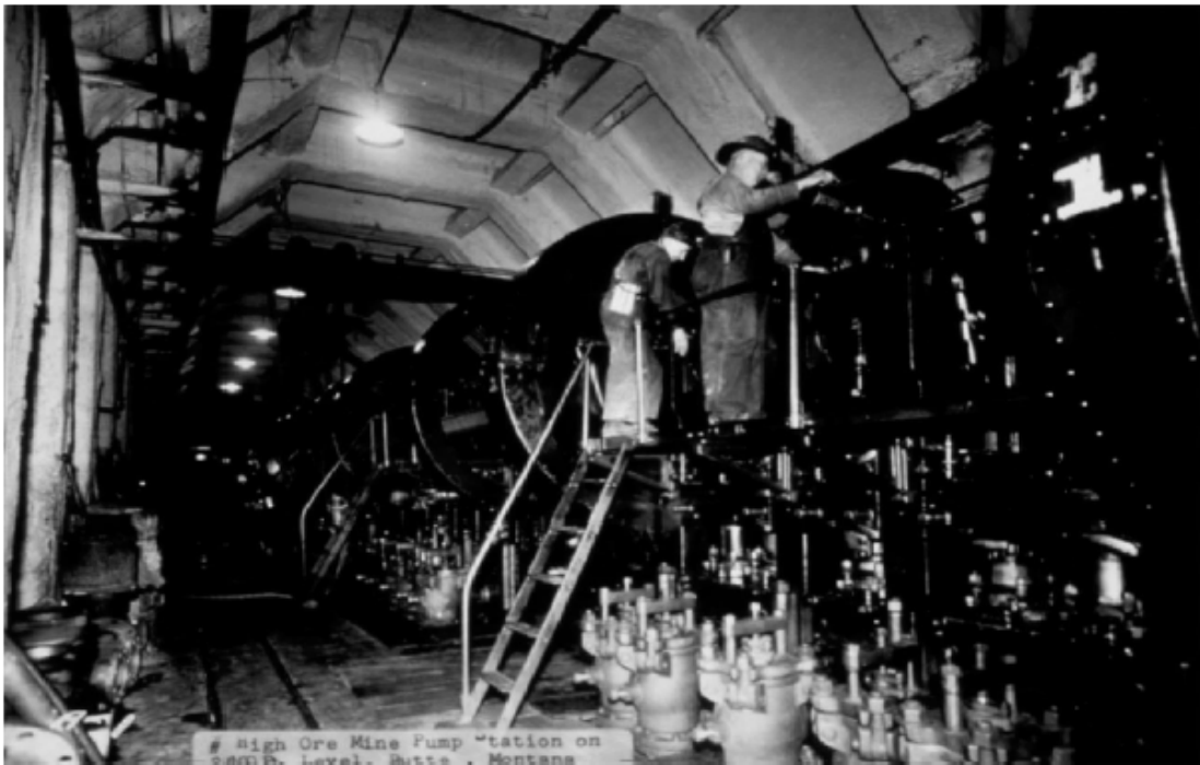
Figure 1-1. High Ore Mine pump station, 2,800-ft level. (Photo courtesy World Museum of Mining, Butte, Montana.)
