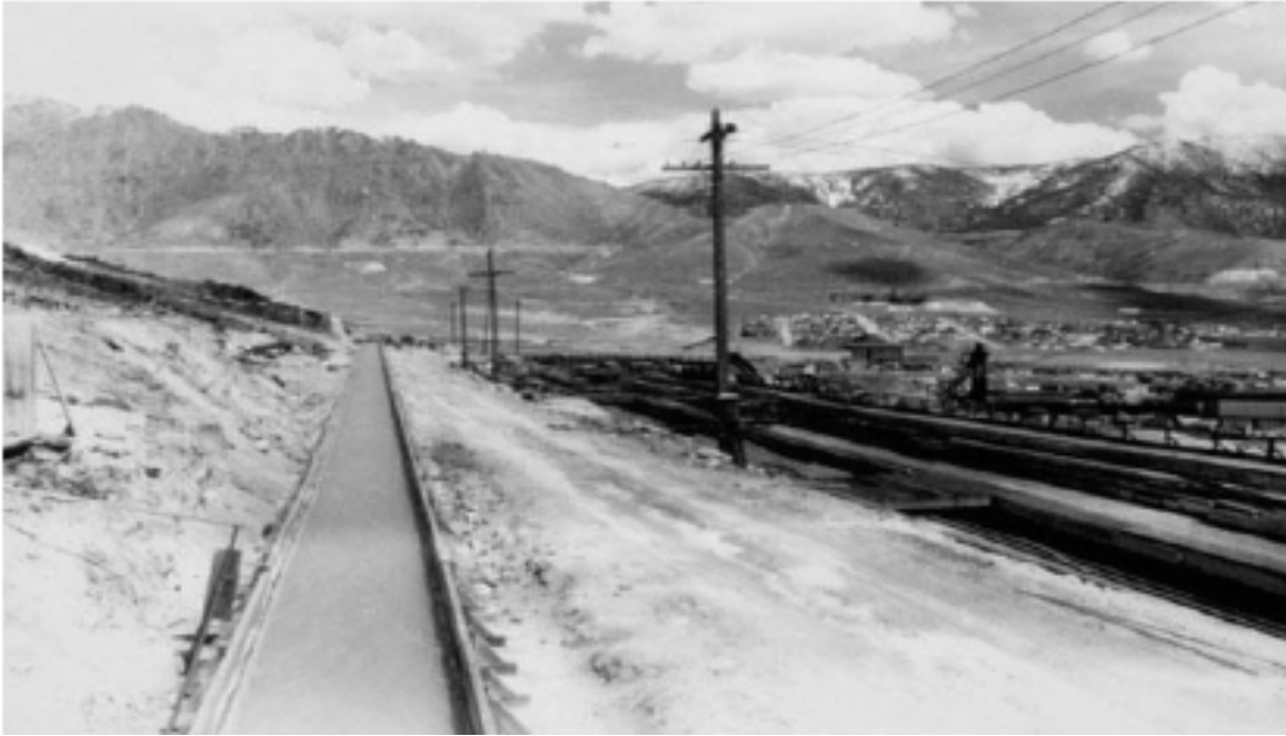
Figure 1-5. Flume conveying water pumped from Butte underground mines to precipitation plant. (Photo courtesy World Museum of Mining, Butte, Montana.)
