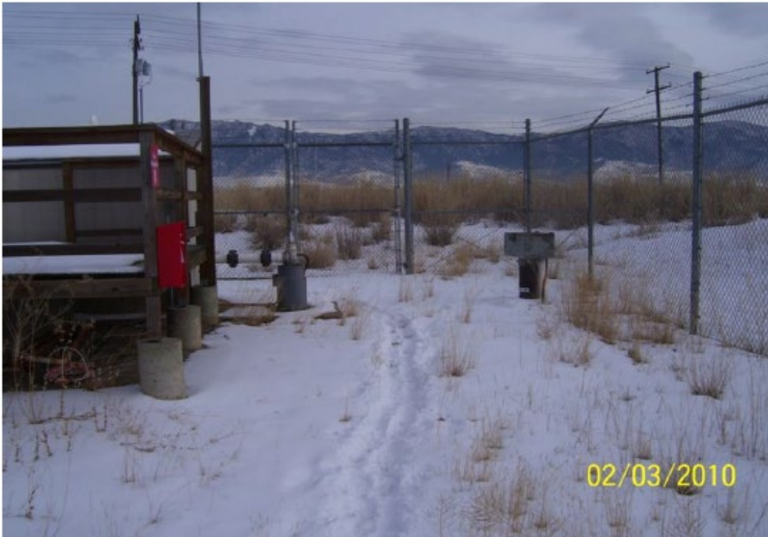
Figure 4-2. West Camp pump station 1997–2011.
