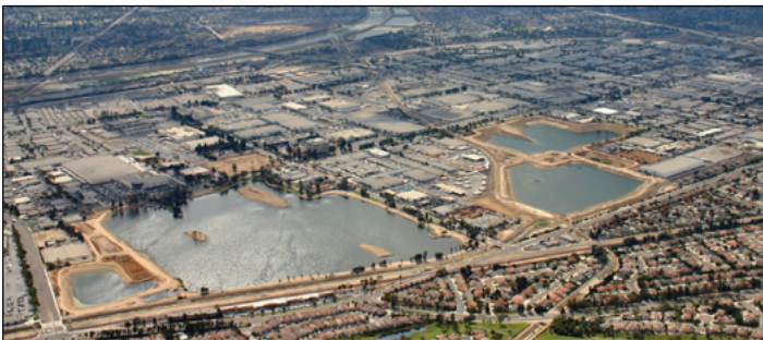
Figure 3. Surface infiltration basins using treated wastewater (source: OCWD, 2024).
