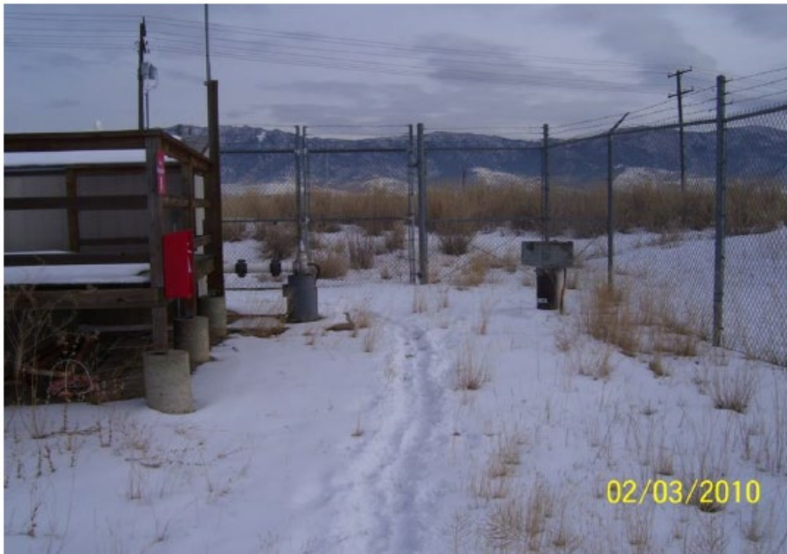
Figure 4-2. West Camp pump station 1997–2011.
