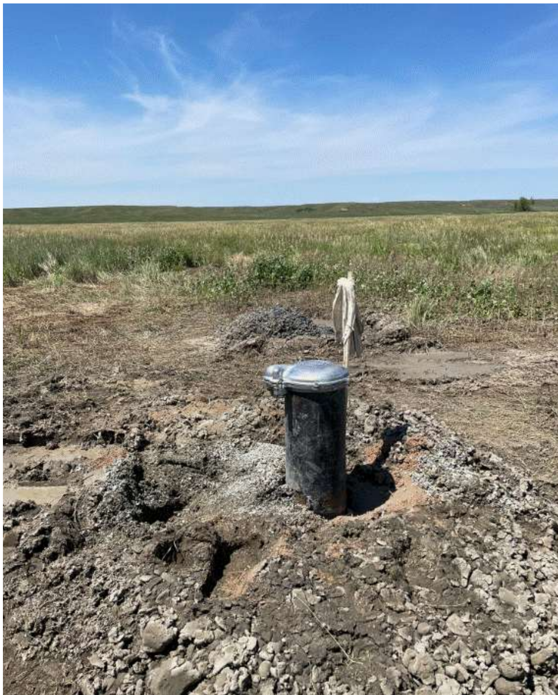
Figure A3. An 8-inch steel protective casing was installed around the PVC monitoring wells.
