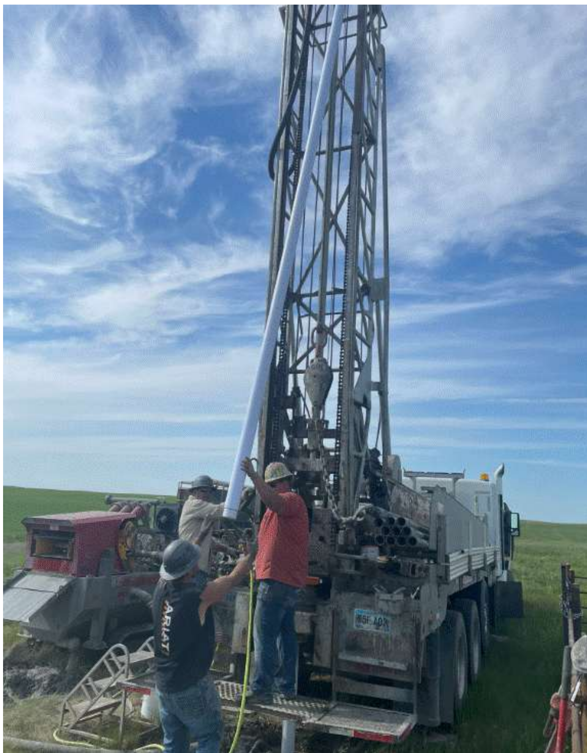
Figure A2. The monitoring wells were constructed with 4-nch PVC casing and factory slotted screen.
