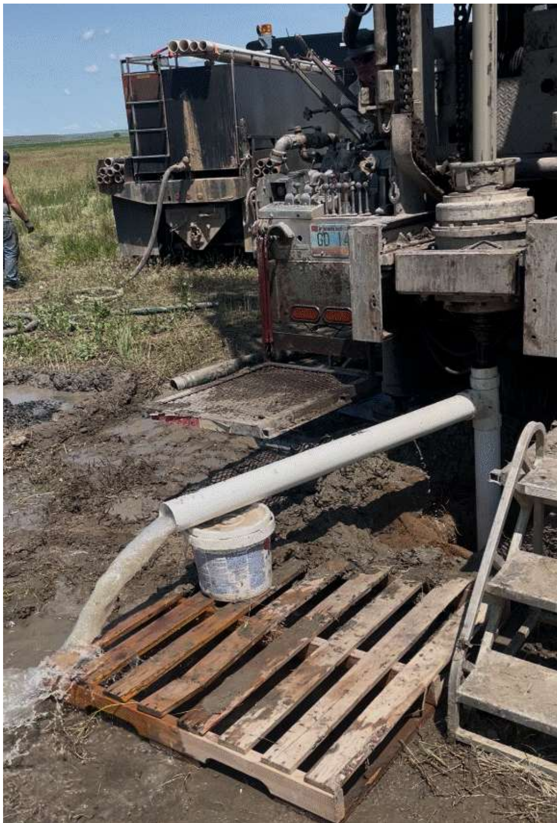
Figure A8. The Big Muddy well (MBMG-338719) produced and estimated 100 gpm during well development.
