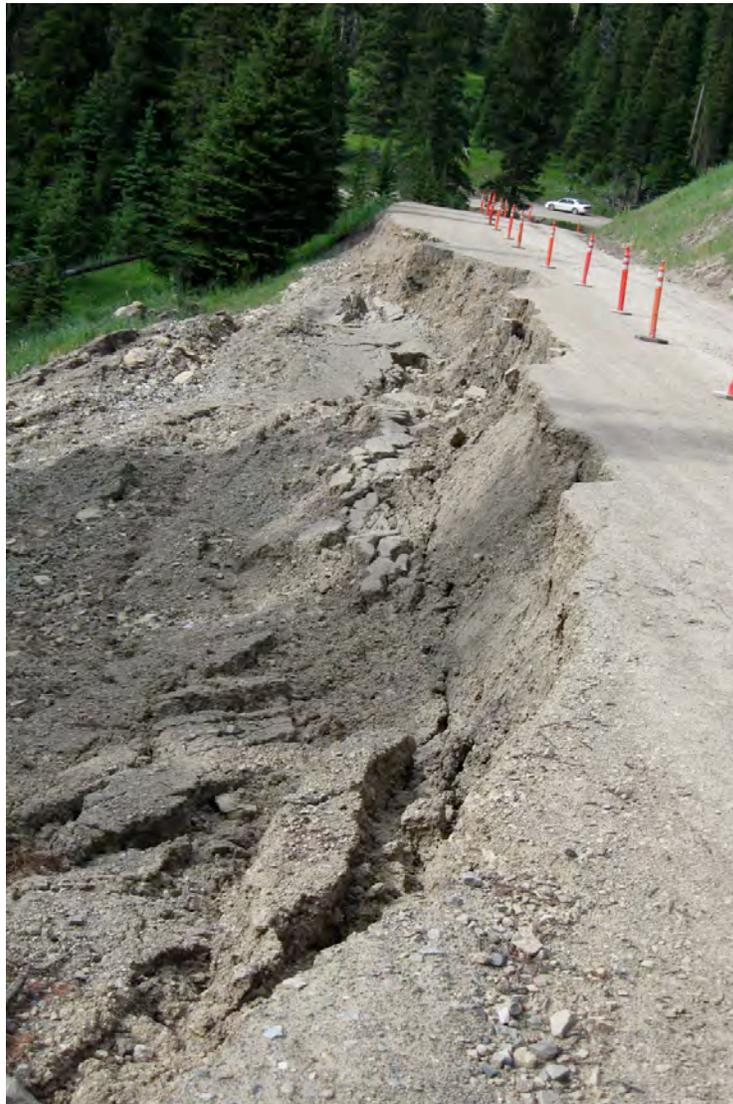
Figure 3. Landslide along Jack Creek Road, promoted by cut-and-fill in an older landslide deposit, coupled with relatively heavy precipitation. Photo taken July 10, 2008.
