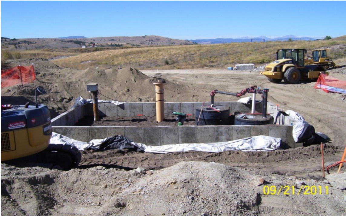
Figure 3-4. West Camp construction of new pump station foundation and infrastructure improvements surrounding pumping well and discharge line.
