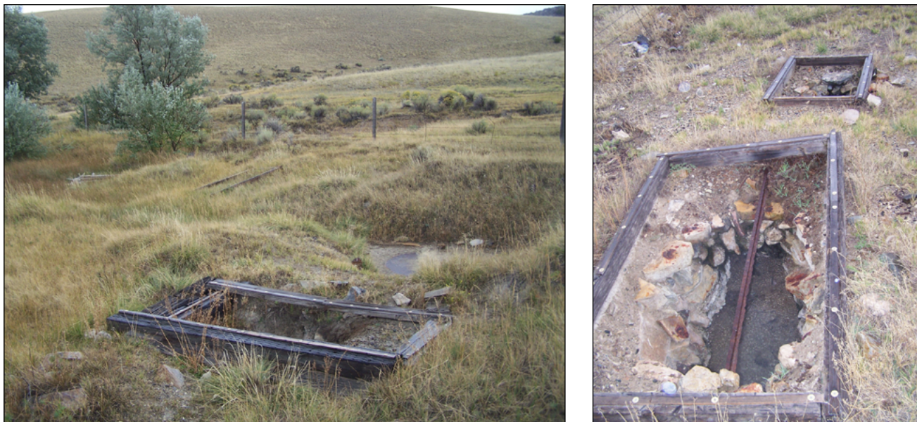
Figure 4. A few of the hot spring vents in Silver Star (note: one spring is covered with a lid, while others are open to the air). Boxes were built around each spring to stabilize the holes. The combined discharge point is located near the trees.
