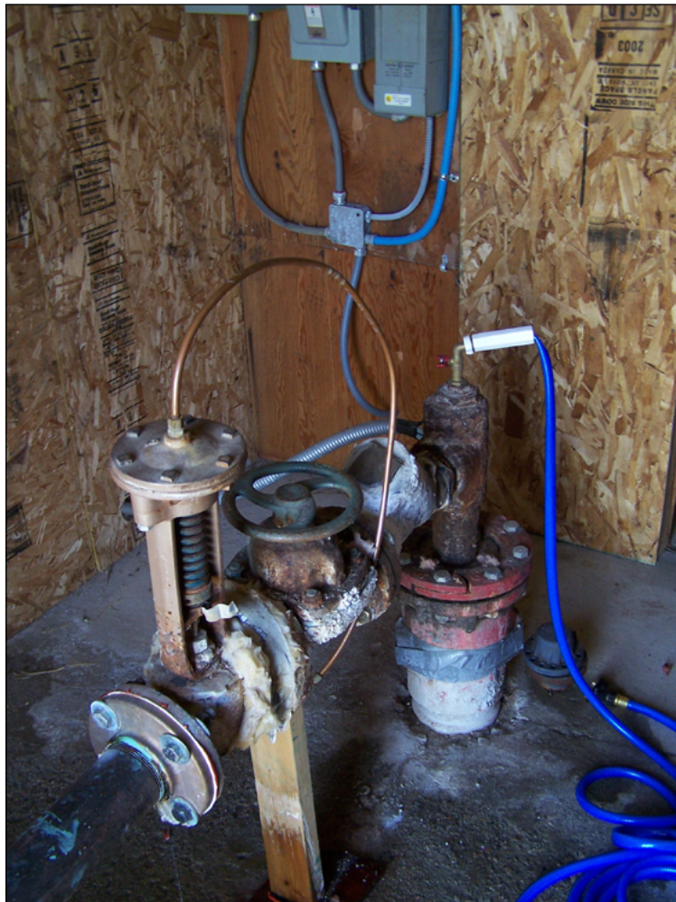
Figure 8. The Fairmont well is located 0.53 km southeast of the resort and springs.
