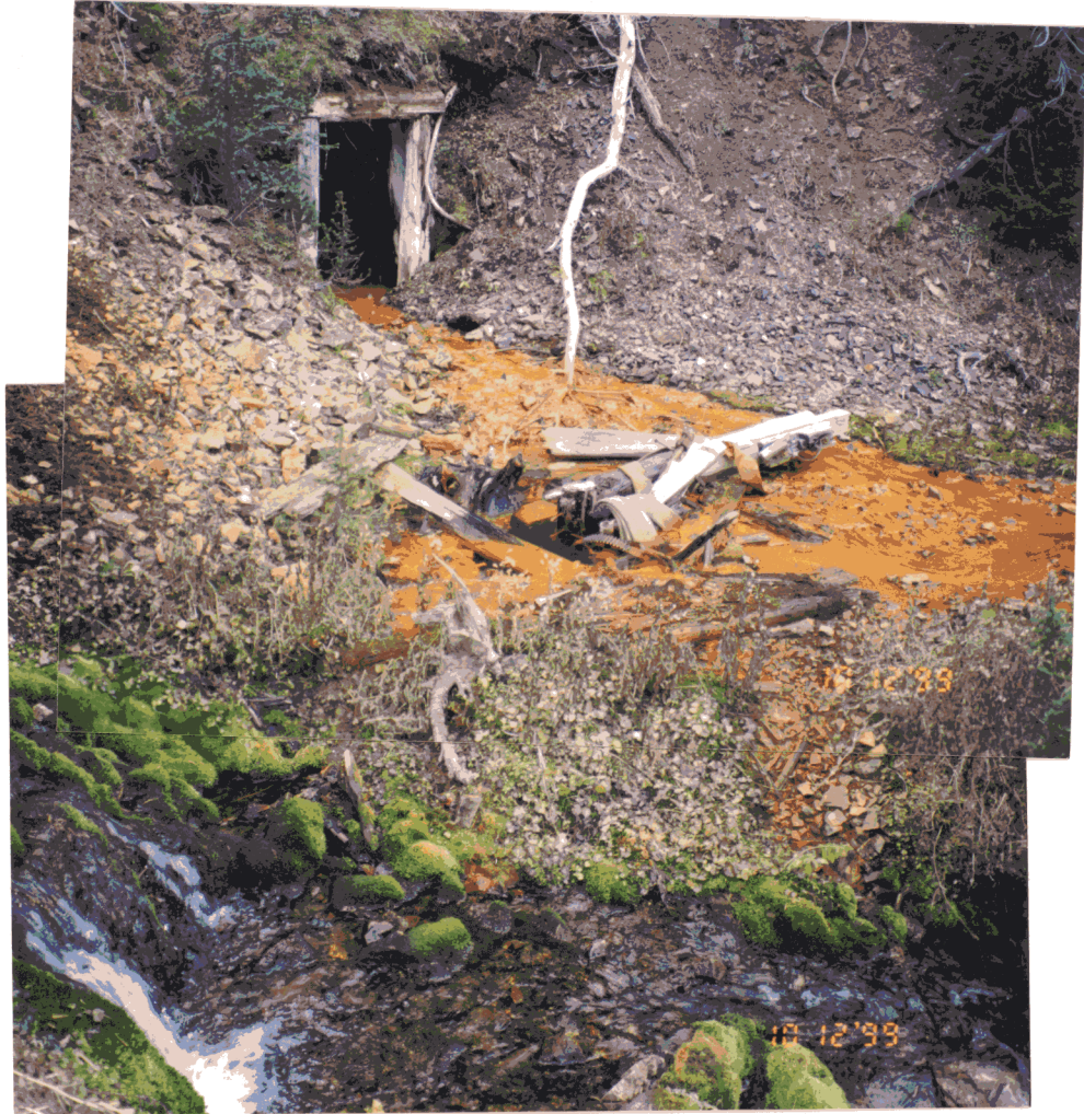
Figure 12b. The flooded shaft and open adit posed physical hazards at the Galena Queen as well as discharging iron-stained water as seen 10/12/99.
