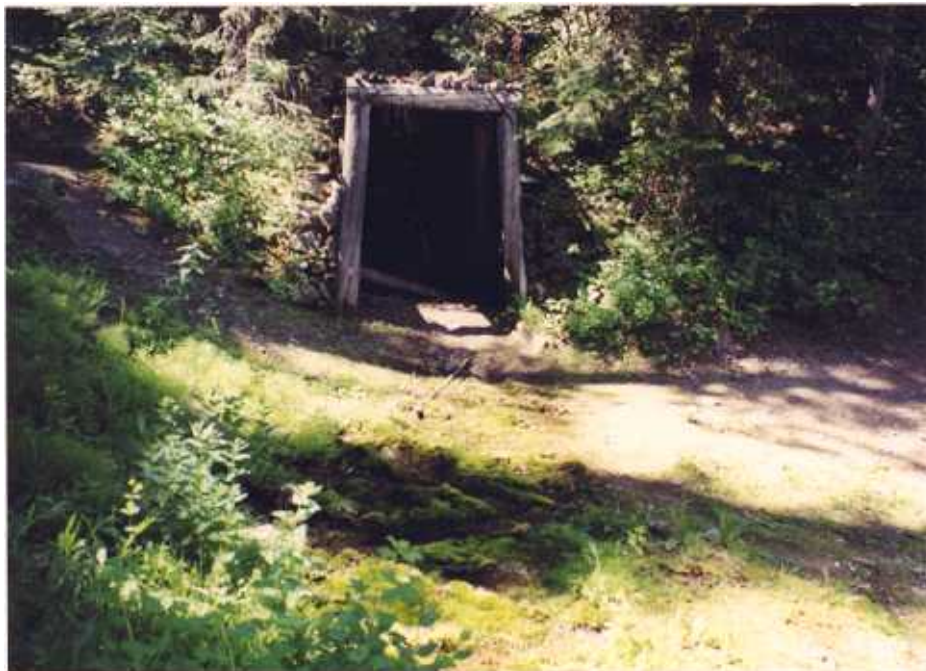
Figure 7b. The lower Johnson Canyon adit was open and a small discharge leaked from in front of the adit and then infiltrated the waste dump.
