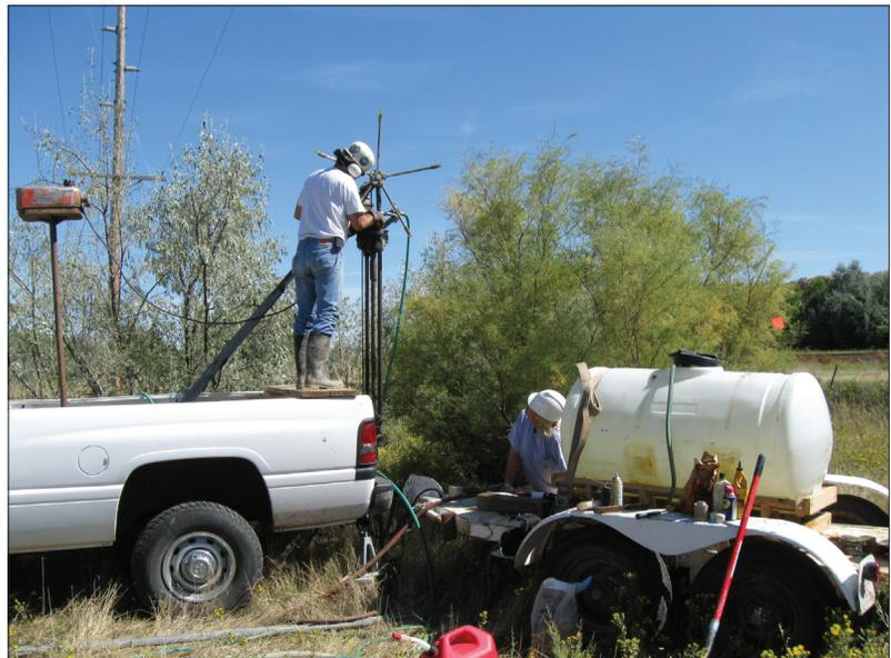
Figure 4. Drilling monitoring wells with a portable Winkey Drill.
