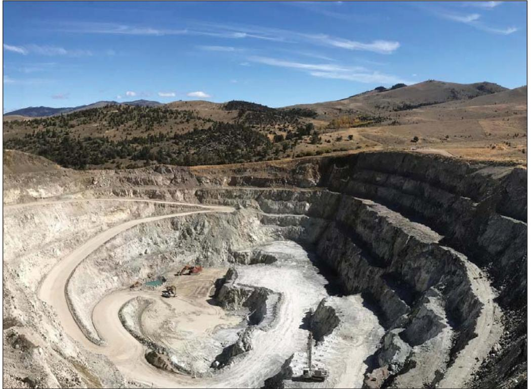
Figure 3. North-facing view of the Regal Mine near Dillon, operated by Barretts Minerals Inc. A permit amendment application was submitted to expand the pit to access additional talc reserves, primarily through deepening and layback of the northern half of the pit.
