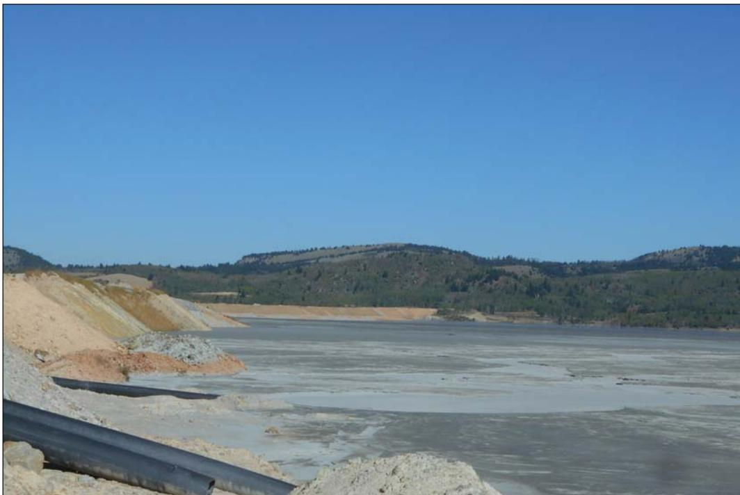
Figure 2. Northwest view across the tailings impoundment at Montana Resources in Butte. An amendment application was submitted to raise the elevation of the west embankment (distant center of photo) and increase the storage capacity of the facility.
