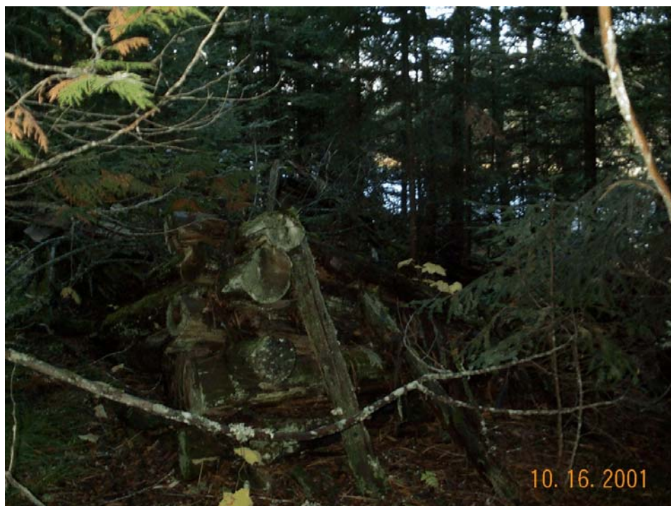
Figure 26a. Stobie-Hermiston Mine had a collapsed cabin that was nearly flattened.
