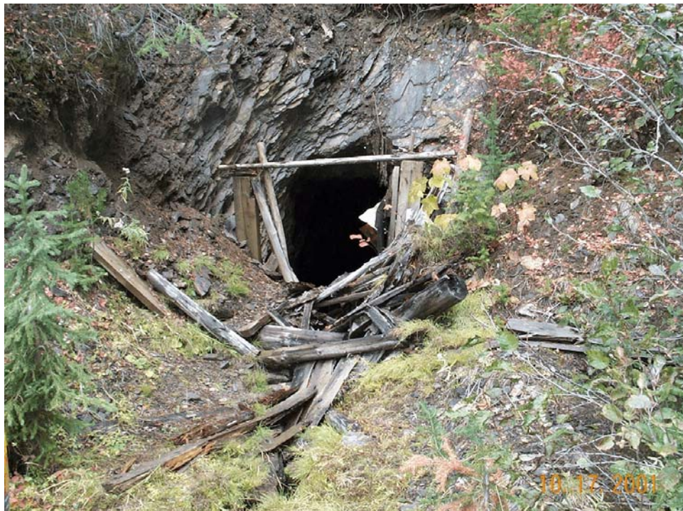
Figure 18b. Adit A01 at the Rock Island Mine was sampled (RRIS20M) where the adit discharged and flowed into the side drainage.
