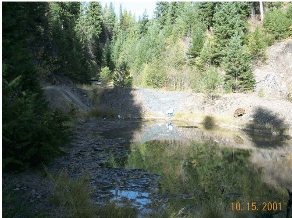
Figure 10b. The Nugget Mine waste rock surrounds a settling pond located downgradient from the discharging adit. Discharge from the pond flows into Kennedy Creek.
