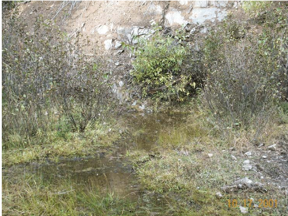
Figure 18a. A possible collapsed adit at the Rock Island Mine was in a marshy area with a seep. The source of the water was uncertain.
