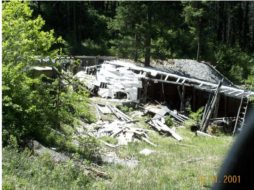
Figure 22c. The Upper Keystone Mine buildings were in poor condition.
