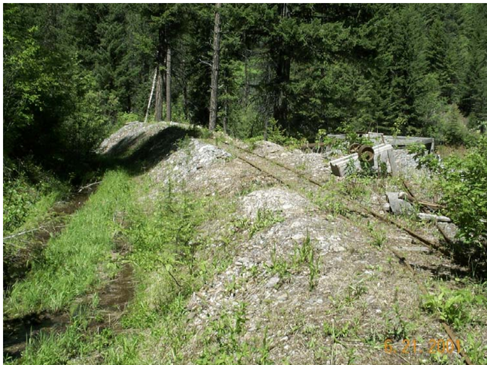
Figure 22b. Upper Keystone Mine waste dump had tracks and an ore bin. The discharge ran along the southwest side of the dump. (Left side in photo.)
