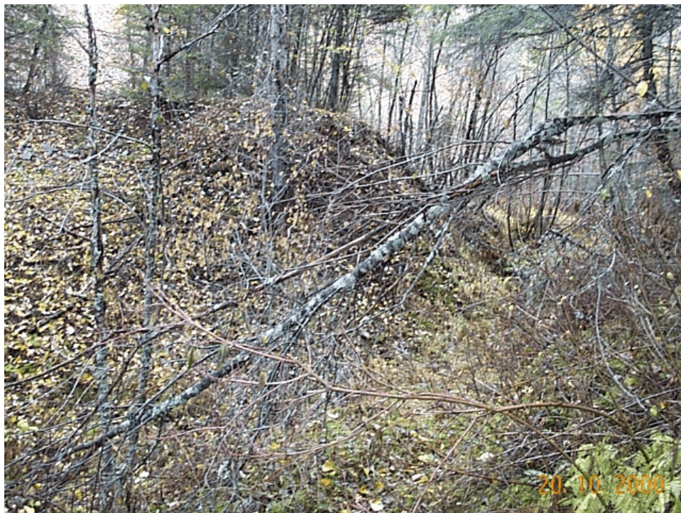
Figure 7b. The tailings-pond dam at the East Fork of Brewster Creek mill site was breached, as mapped on 10/20/00.
