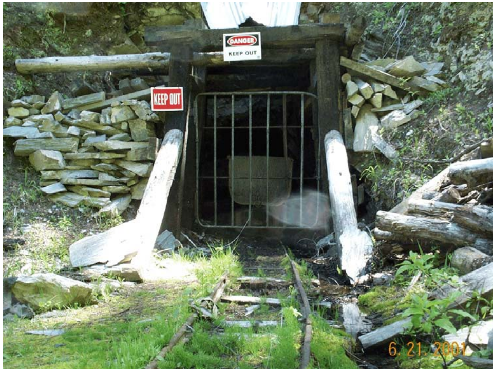
Figure 22a. The Upper Keystone Mine adit was open but had a locked gate when visited on 06/21/01.
