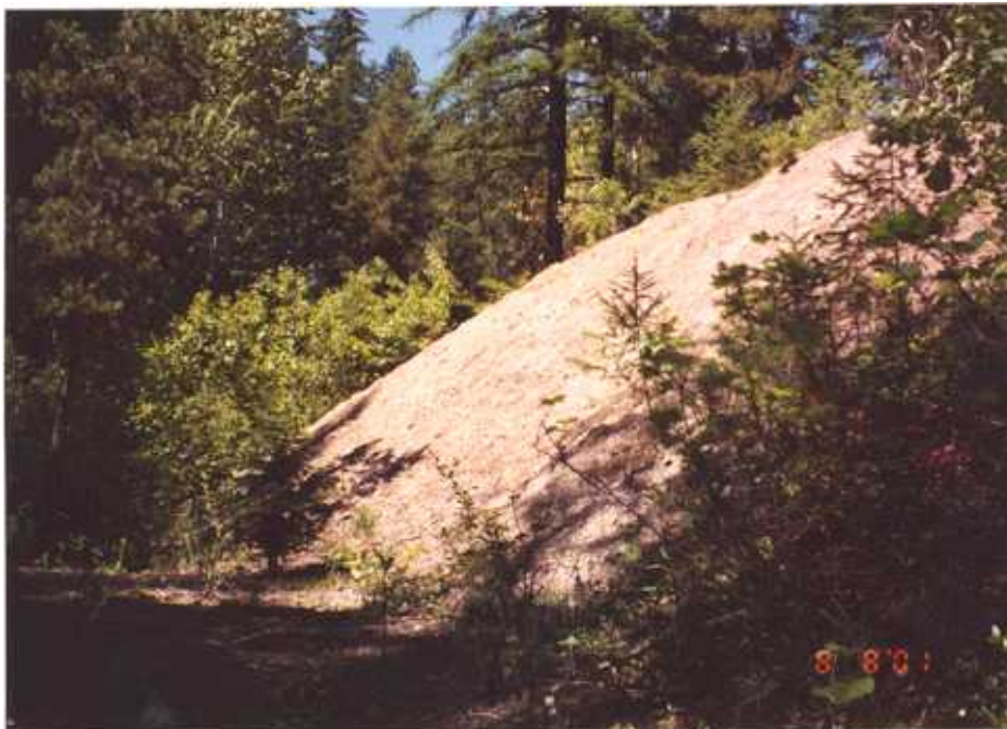
Figure 13b. The Last Chance waste dump had a low probability of failure on most slopes but was being undercut on the east side by Last Chance Creek.
