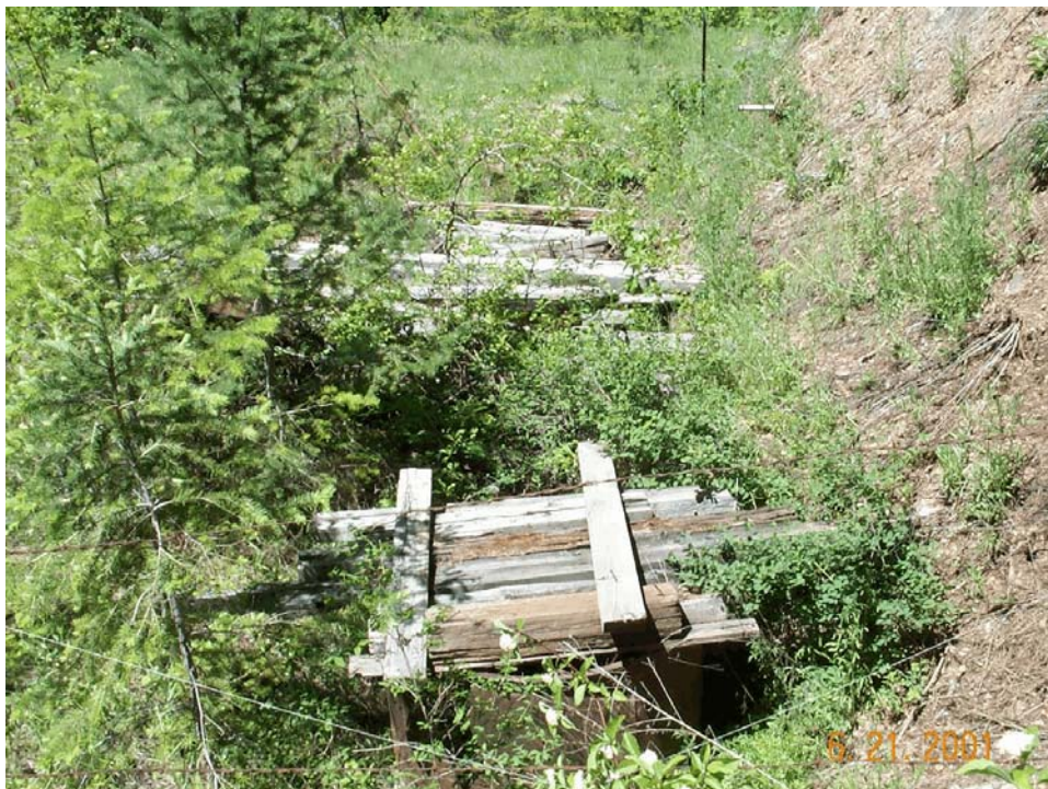
Figure 22d. The Upper Keystone Mine had a fenced structure, perhaps a shaft.
