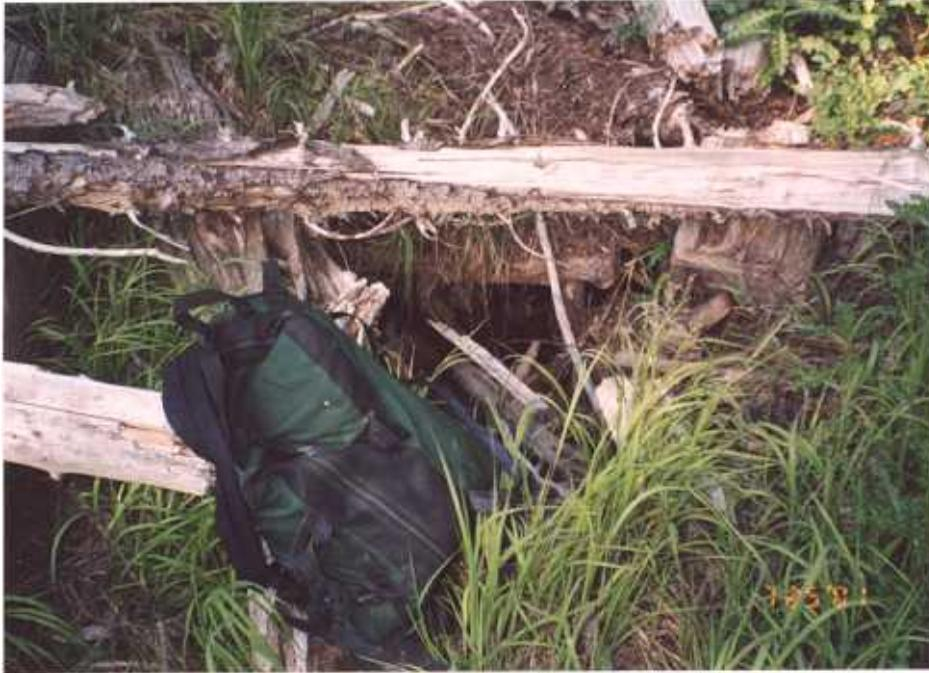
**Figure 21a.** One of the dry adits near Crystal Lake was almost entirely obliterated with only a few timbers showing.
