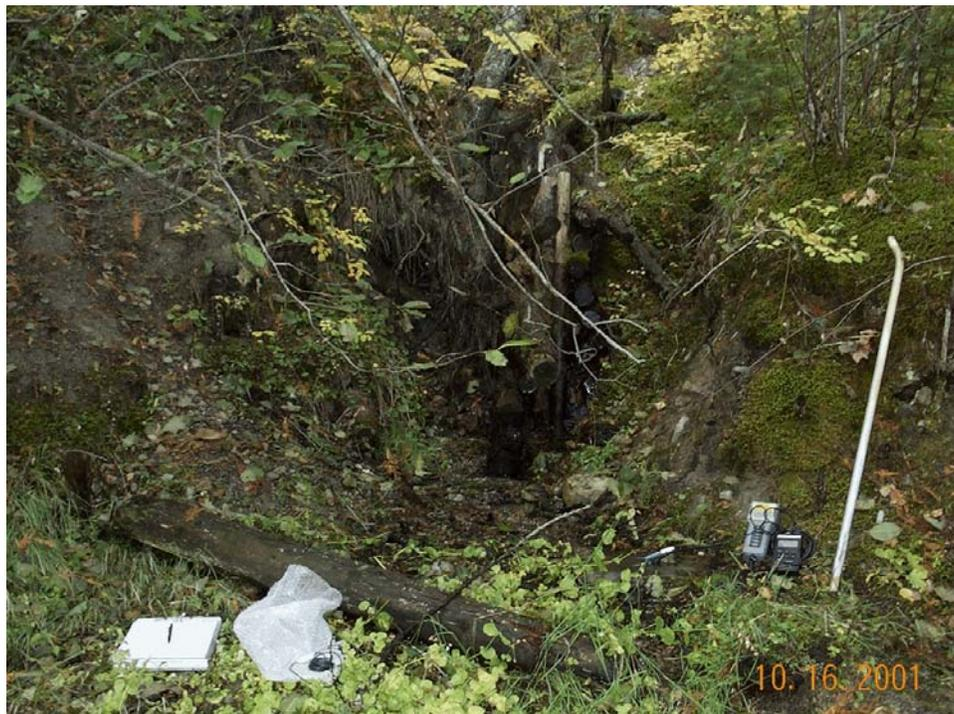
**Figure 26b.** The Stobie-Hermiston Mine's adit discharge flowed over the waste-rock dump and down toward the Clark Fork River.
