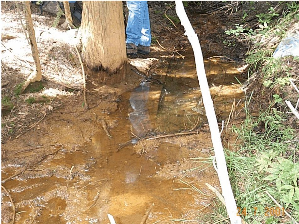
**Figure 24a.** Discharge from the Vulcan Tunnel emerged from a collapsed adit and ponded in front of the portal.
