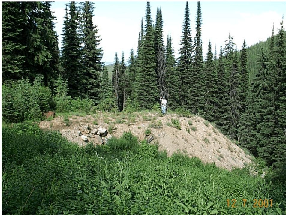
**Figure 20d.** Big Sunday Mine waste-rock dump was uphill from Big Sunday Creek. The adit discharge was to the left in the photo and infiltrated into the waste rock.
