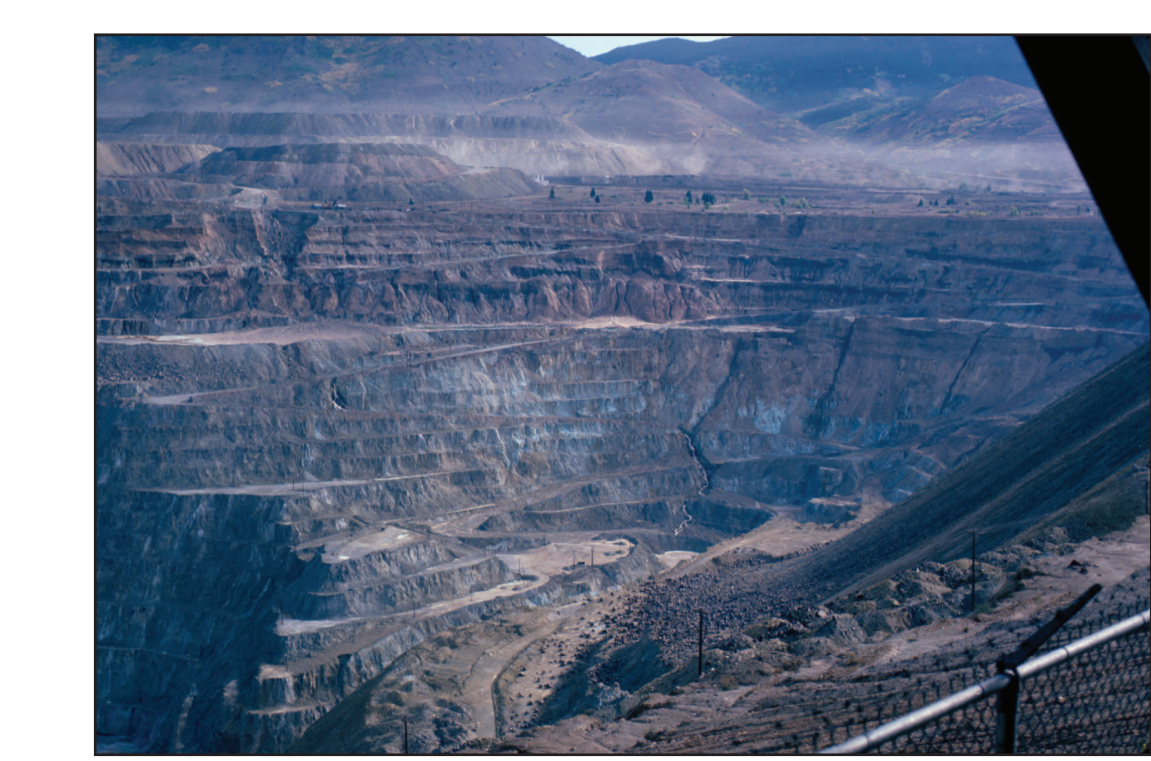
Figure 3. View looking northeast showing erosion of pit haul roads from surface-water discharge, September 1984.
