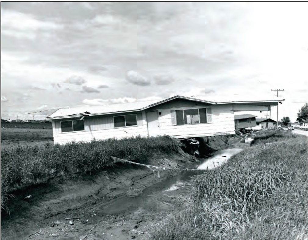
Homes and buildings damaged during Teton Dam failure
