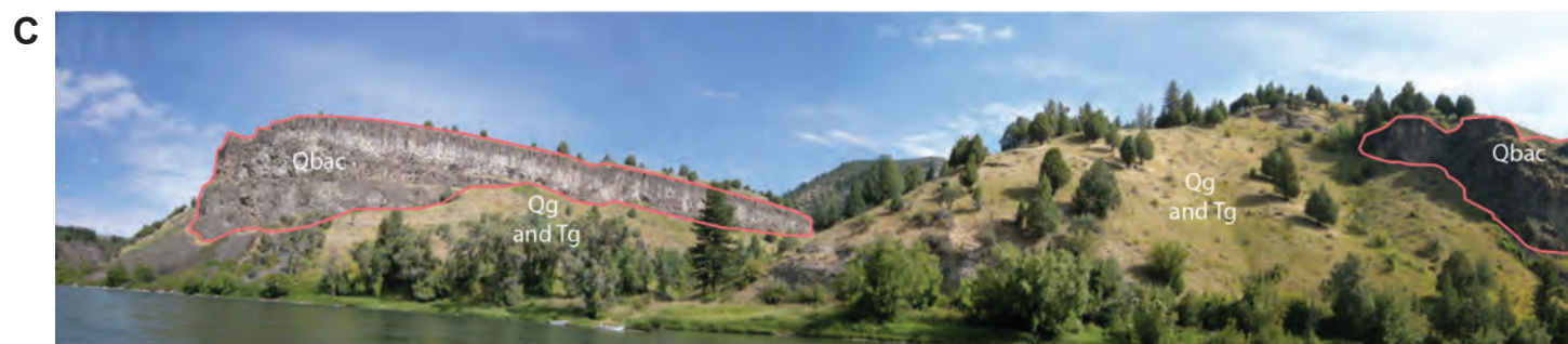
Figure 7. Ancient canyon walls. A-C. Annotated images showing the distribution of the paleocanyon-fill facies of the basalt of Antelope Flat (Qbac) at Dry Canyon (A; Location I in fig. 1), Pine Creek Canyon (B; Location J in fig. 1), and Gomer Canyon (C; location K in fig. 1); Qbar is the plateau facies; Qyh is the Huckleberry Ridge Tuff; Qg and Tg are gravel; PMu are Paleozoic sedimentary rock units. The basalt is thick where it flowed into and partially filled the canyons and thins rapidly up canyon walls and into tributary canyons.
