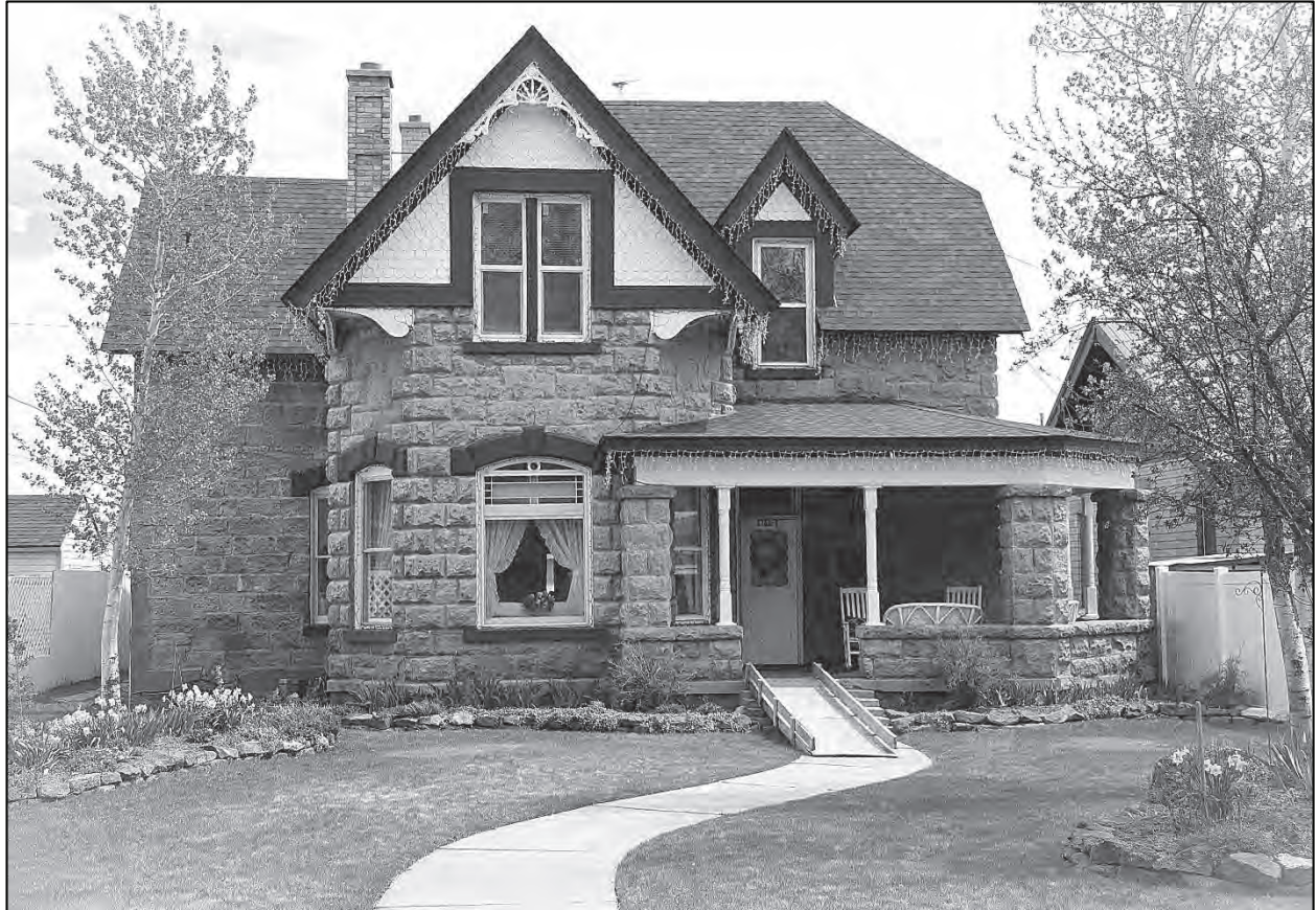
Earliest Stone House in Rexburg: John Smalley and Tamera Ricks built this home in 1892 from blocks of Huckleberry Ridge Tuff. Today it lies at at 112 N 1 st E Street in Rexburg. Like most local stone buildings, the 24-inch-thick exterior walls withstood the Teton Flood waters far better than modern frame and brick houses. (Photo courtesy of Glenn Embree.)
