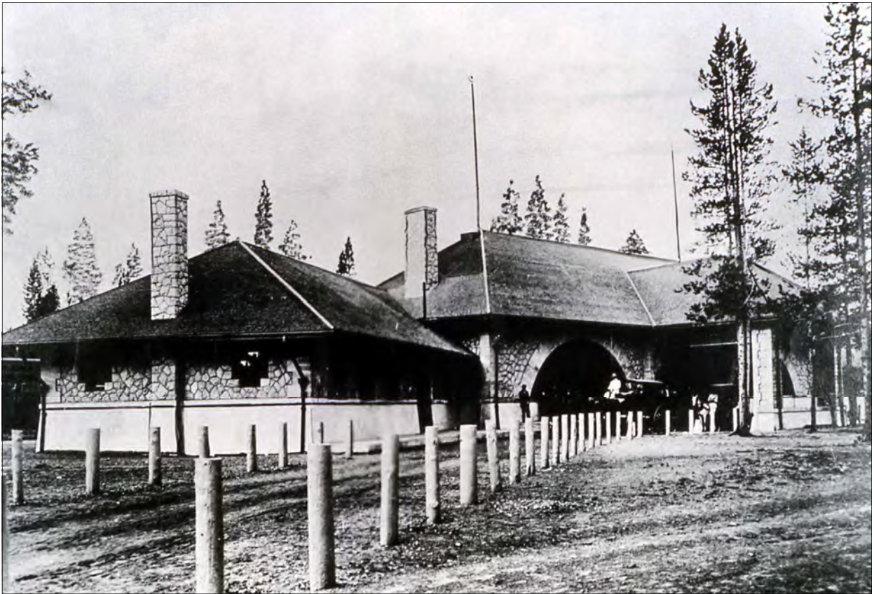
Oregon Short Line depot at West Yellowstone, about 1908. Courtesy National Park Service.
