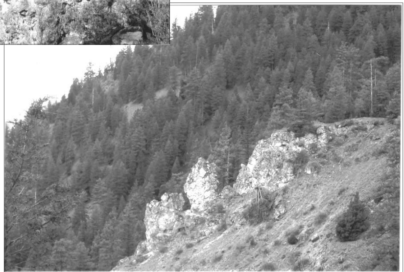
Figure 4 - Knobs of brecciated dolomite near the headwall of the Alberton landslide. The middle knob is ~20 ft high, view is northwest. The forested hill-slope on the skyline is underlain by Helena Formation argillite and siltstone.
