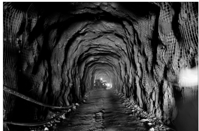
Figure 7. View down the exploration decline, Butte Highlands Gold Project.
