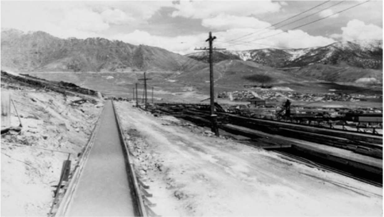
Figure 1-4. Flume conveying water pumped from Butte underground mines to precipitation plant. (Photo courtesy World Museum of Mining, Butte, MT.)
