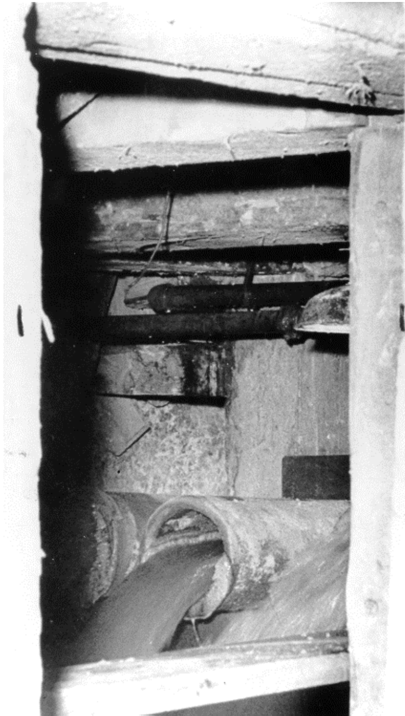
Figure 1-3. Underground mine drainage from Belmont Mine to High Ore Mine. (Photo courtesy World Museum of Mining, Butte, MT.)
