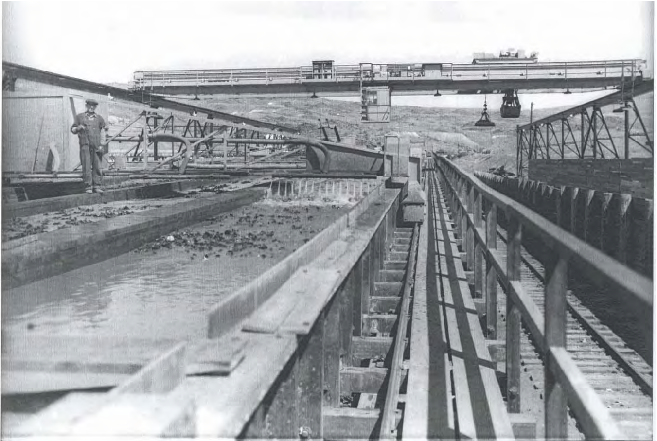
Figure 1-5. Precipitation plant scrap iron in contact with underground mine discharge water. (Photo courtesy World Museum of Mining, Butte, MT.)
