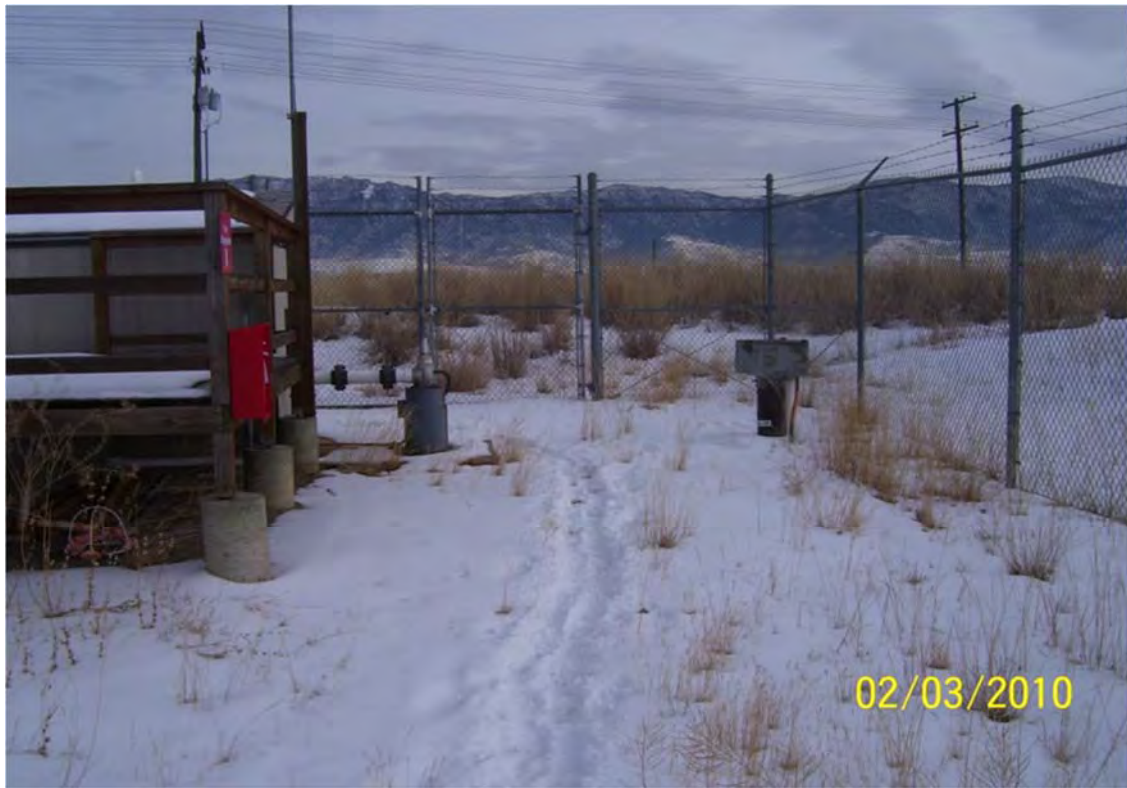
Figure 4-2. West Camp pump station 1997–2011.
