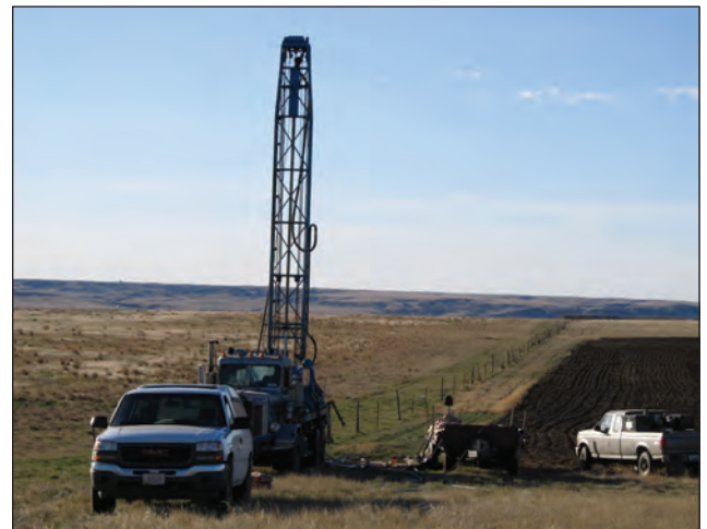
Figure 6. Monitoring well installation north of Burns Creek.
