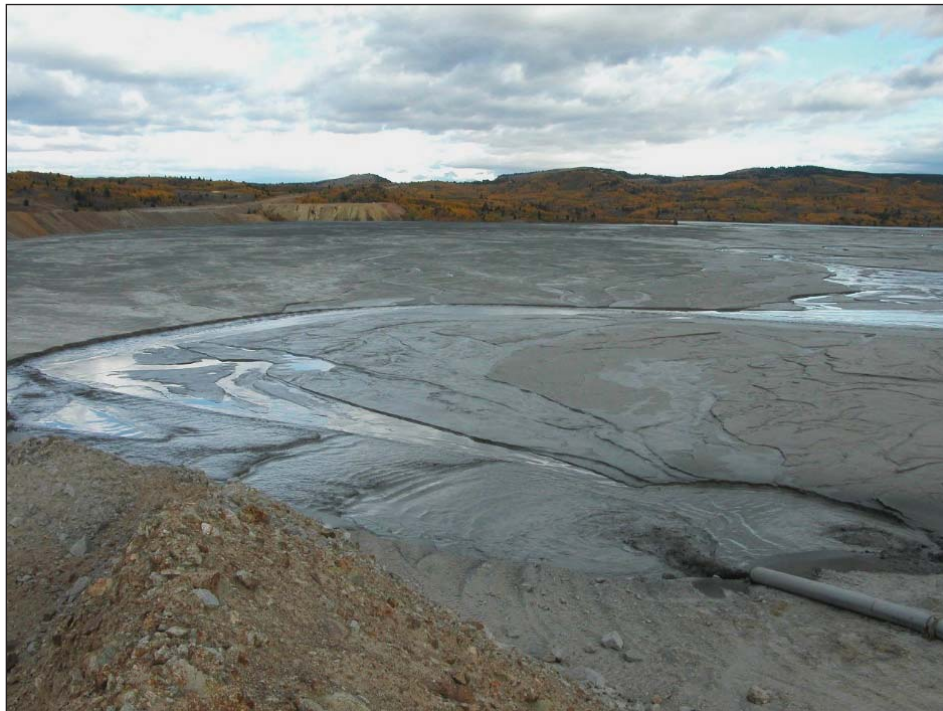
Figure 10. Approximately 18,000 gallons per minute (1,130 L/sec) of mill tailings are discharged as a slurry (40% solids) into the Yankee Doodle impoundment (photo taken in October 2005).
