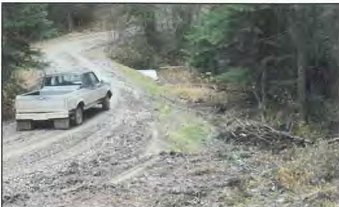
One of the most common road drainage problems is allowing ditch drainage to flow directly into a stream. Always route ditch drainage through a filter (vegetated buffer zone, slash filter windrow) to remove sediment from the water before it reaches the stream.
