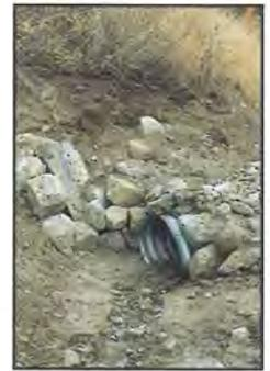
Drop inlets (left photo) installed at the head of a ditch relief culvert below the flow of water help settle out sediment and prevent the culvert from plugging. Rock armored inlets prevent water from eroding and undercutting the culvert and flowing beneath the road.
