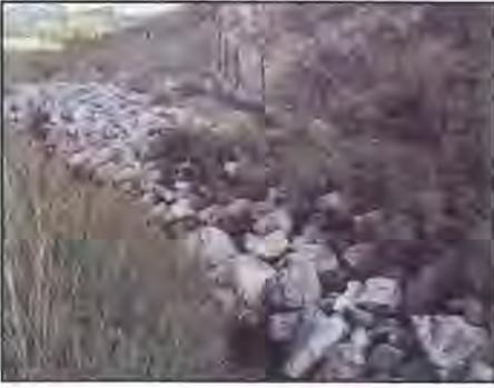
Place riprap in diversion ditches to prevent ditch erosion and subsequent failure.
