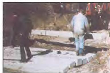
Plan for flood (25 yr/6 hr storm event) conveyance. An improperly sized crossing will result in erosion and potential loss of the structure. When future floods are ignored, the potential for water-quality damage is enormous. Usually, costs of repair far exceed costs of proper installation.
