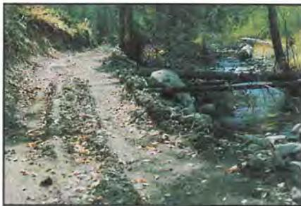
If grading produces excess material, feather it out or haul it away. **Never side-cast material into streams.** Avoid leaving a berm that channels water down the road unless it is routed into an effective vegetation filter which spreads it out and removes sediment.
