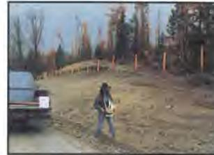
Grass seeding on raw, exposed cut-and-fill surfaces is an important erosion control practice. Exact seed mixtures, proper timing, and fertilizers are important for success. Seed as soon as possible after dirt work is completed.
