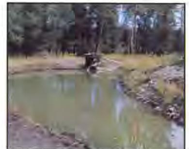
Direct ground water from dewatering operations and runoff from disturbed lands to the settling pond.
