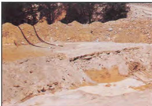
Clean settling ponds. Containment berms should be stabilized with enough freeboard to allow for spring runoff and snowmelt.
