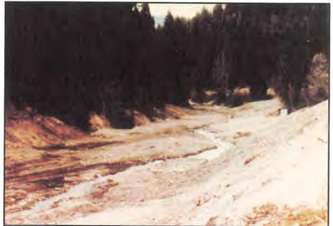
Regrading of mine site and reestablishment of stream channel and flood plain.
