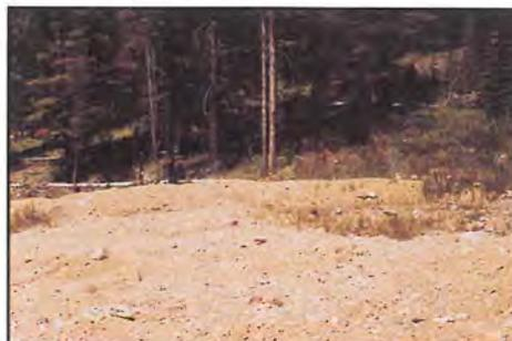
Construct and stabilize diversion berms to divert spring runoff and snowmelt.
