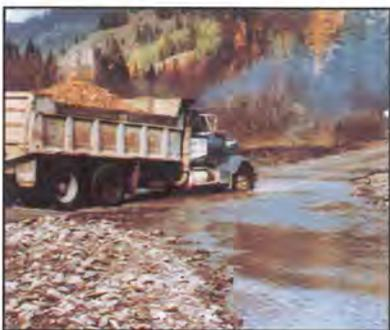
Limited traffic on this improved ford crossing has minimal impact on the streambed and produces little sediment.
