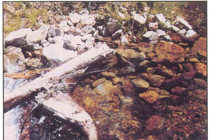
Construct pools (energy dissipators) with rocks or boulders to reintroduce the channelized flow into the existing stream below the mine area.
