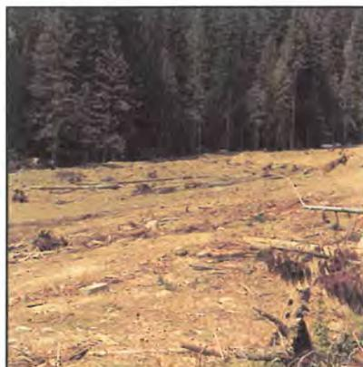
**Spread brush and slash** from clearing operations on reclaimed ground to trap sediment being transported to live streams and protect new vegetation. To effectively control erosion, the slash must touch the soil surface.
