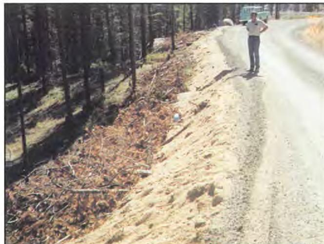
Slash filter windrows are very effective at keeping sediment from entering stream channels. They commonly measure 3 x 3 feet and consist of compacted slash installed along the base of the fill slope.
