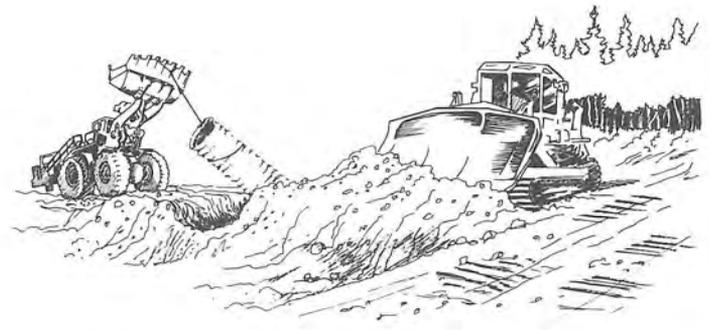
If you decide to remove bridges and pull all culverts, you must restore all drainage features to their natural condition. This includes recontouring and reseeding all disturbed surfaces.
