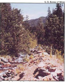
Riprap drains and diversions with cobbles and boulders. Place riprap in areas which may erode during high flows.
