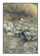
Drop inlets (left photo) installed at the head of a ditch relief culvert below the flow of water help settle out sediment and prevent the culvert from plugging. Rock armored inlets prevent water from eroding and undercutting the culvert and flowing beneath the road.
