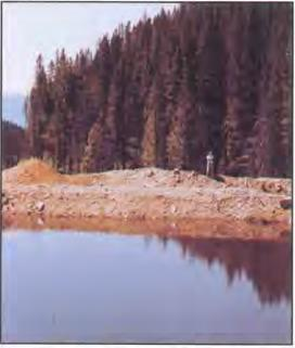
Silt pond dike showing adequate freeboard.
