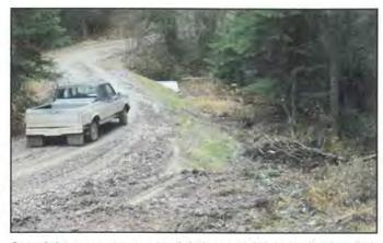
One of the most common road drainage problems is allowing ditch drainage to flow directly into a stream. Always route ditch drainage through a filter (vegetated buffer zone, slash filter windrow) to remove sediment from the water before it reaches the stream.
