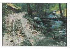
If grading produces excess material, feather it out or haul it away. Never side-cast material into streams. Avoid leaving a berm that channels water down the road unless it is routed into an effective vegetation filter which spreads it out and removes sediment.
