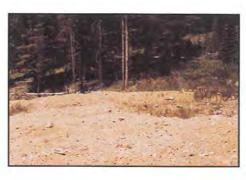
Construct and stabilize diversion berms to divert spring runoff and snowmelt.
