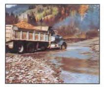
Limited traffic on this improved ford crossing has minimal impact on the streambed and produces little sediment.
