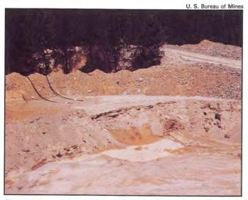
**Clean settling ponds** daily to weekly depending on design. The ponds should never be more than 50 percent full of sand, gravel, or silt.
