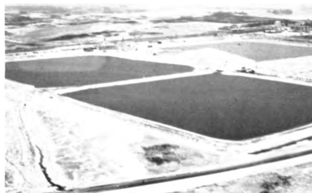
Figure 2-5.—The three Chaplin Lake reservoirs, which have a 300-million-gallon brine storage capacity.
