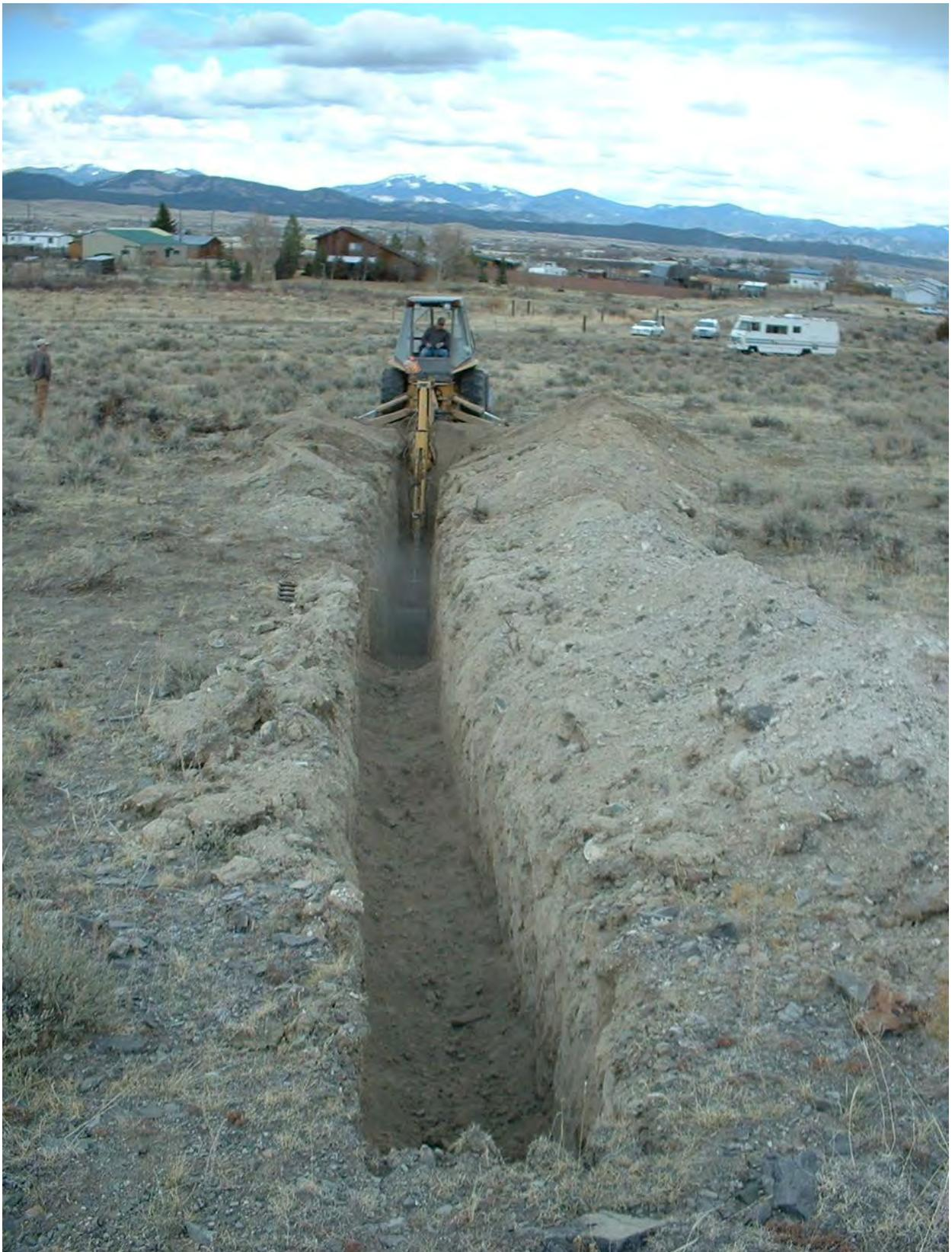
**Figure 9.** Excavation of southern trench. Note the darker color of the excavated material just in front of the backhoe where younger alluvial fan material was encountered.
