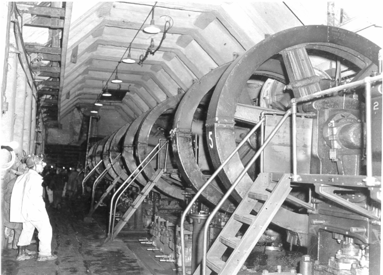
Figure 1-1a. High Ore Mine pump station located on the 2800 level. (Photo courtesy of the World Museum of Mining.)
