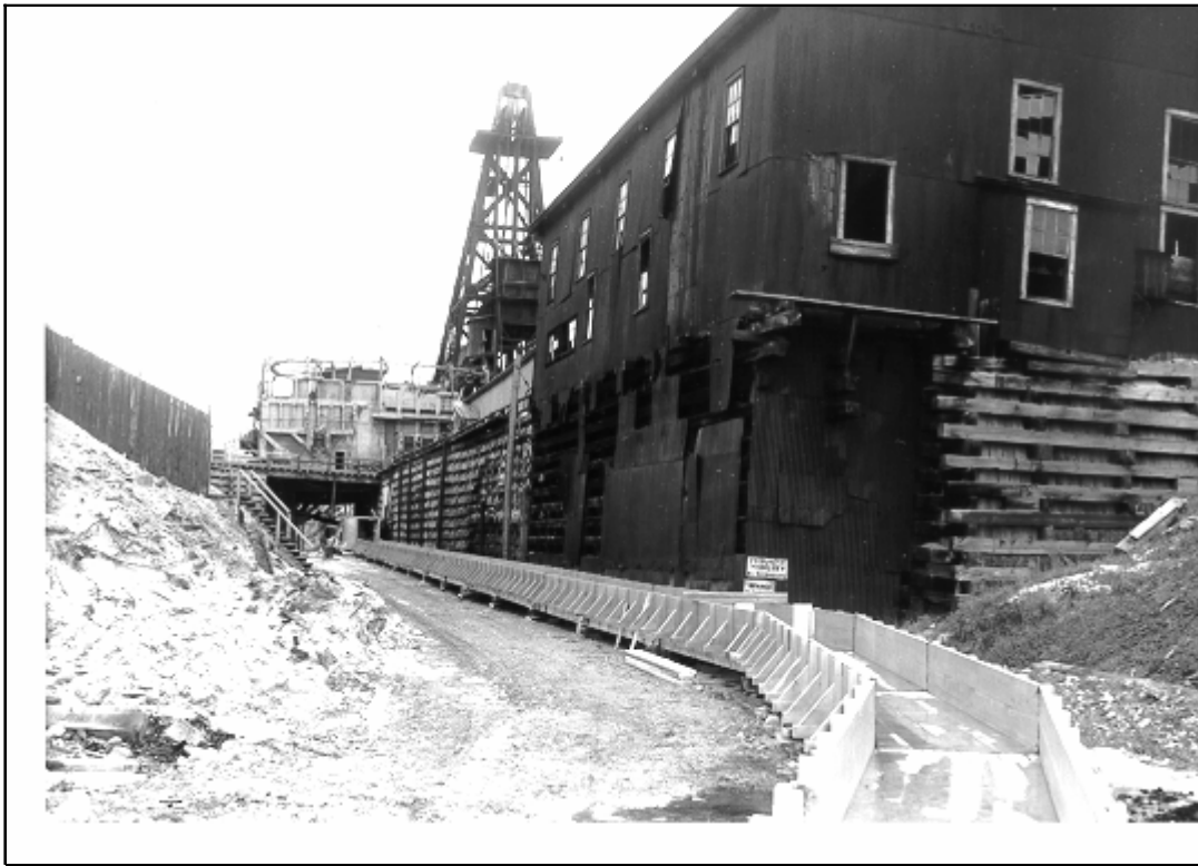
Figure 1-1. Flume used to carry underground mine water pumped from the High Ore mine pump station to the precipitation plant for leaching of copper from the water.
