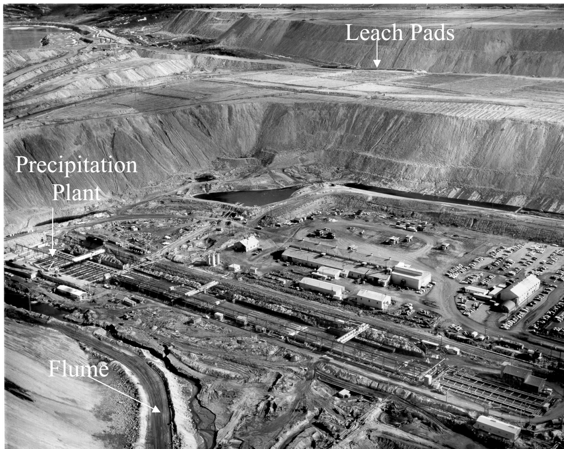
Figure 1-1. Photo showing precipitation plant, leach pads, and flume carrying water from underground mines.
