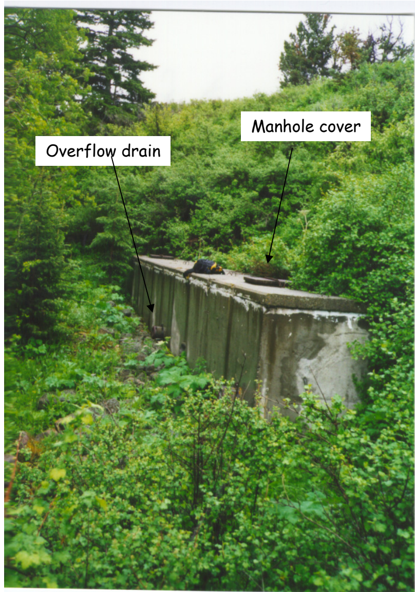
Photo 1. Upper spring box (source #003), looking southwest. Slope of glacial moraine is behind the spring, Bear Creek is immediately to the left. View shows manhole covers on top of box and overflow pipe in lower center portion of the spring box side.
