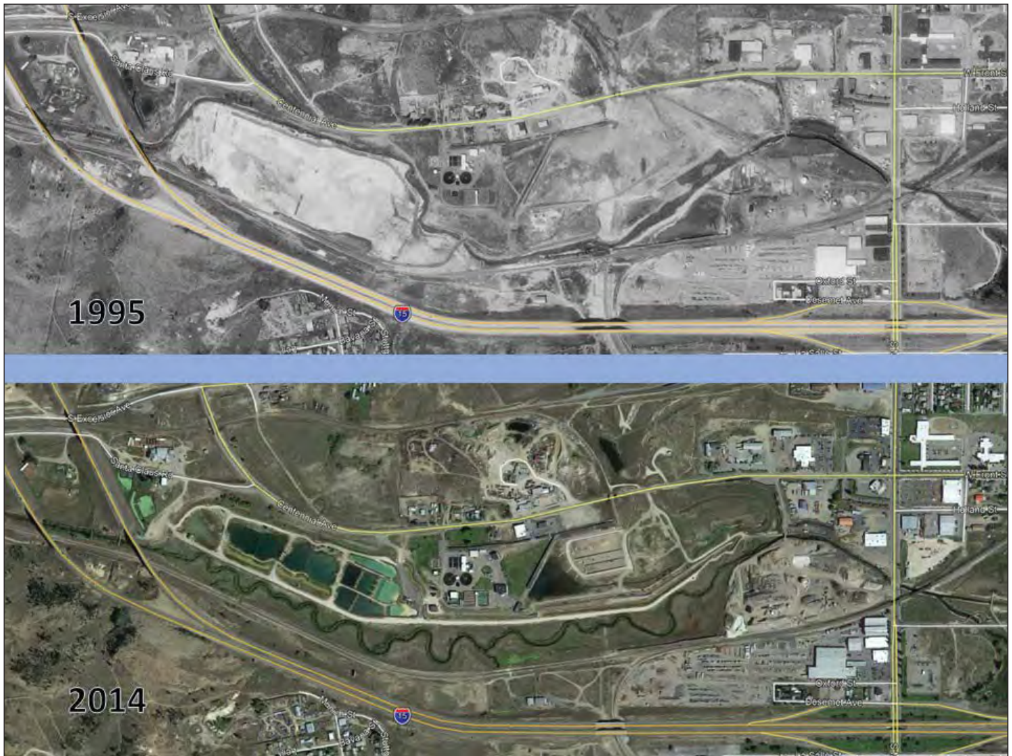
Figure 2. Google Earth images, before and after the environmental cleanup of the Colorado Tailings/Butte Reduction Works (CT/BRW) area. The CT is the rectangular light gray area on left with SBC outlining the northern boundary. In the post-reclamation image, SBC and its floodplain have been reconstructed to the south of its original location. The Butte Treatment Lagoons are a lime addition groundwater treatment system located at the former CT. The two circular clarifier tanks mark the Butte Sewage Treatment Plant.
