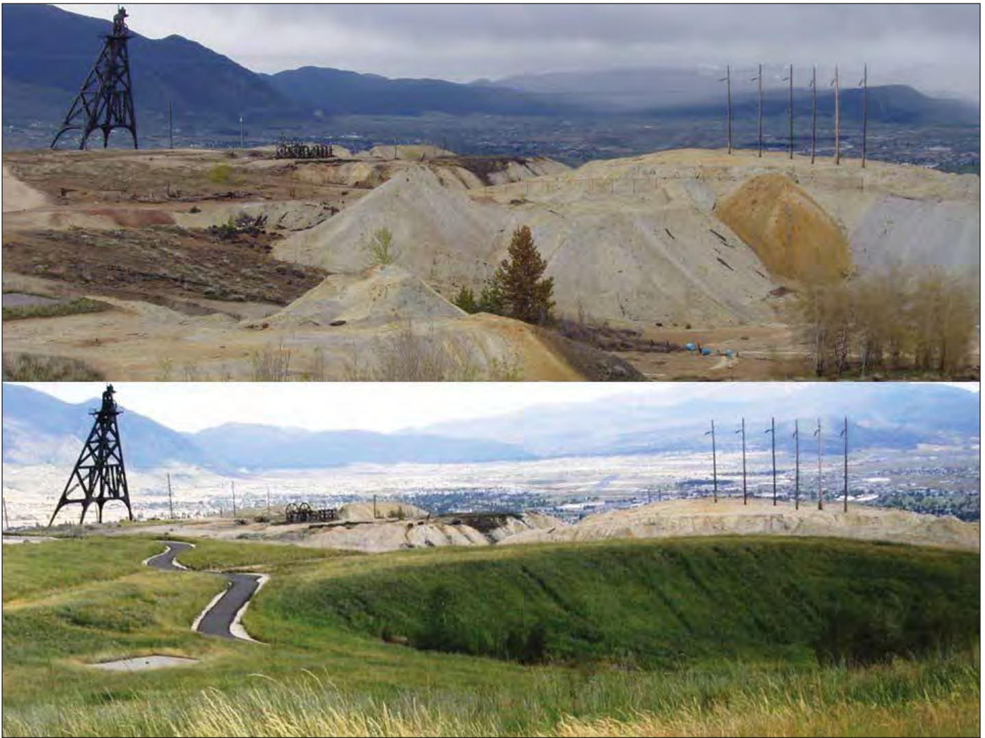
Figure 3. Before and after photographs of mine dump reclamation. The Diamond mine is marked by the prominent headframe.
