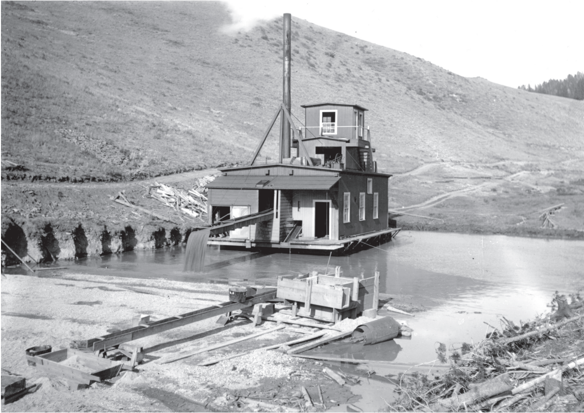
Figure 11. One-cubic-foot bucket-line dredge of the Variegated Sapphire Company, built and operated by members of the Dodd family on the South Fork of Dry Cottonwood Creek above Grand Pre Flat. Photo by Douglas B. Sterrett, U.S. Geological Survey, June, 1910.
