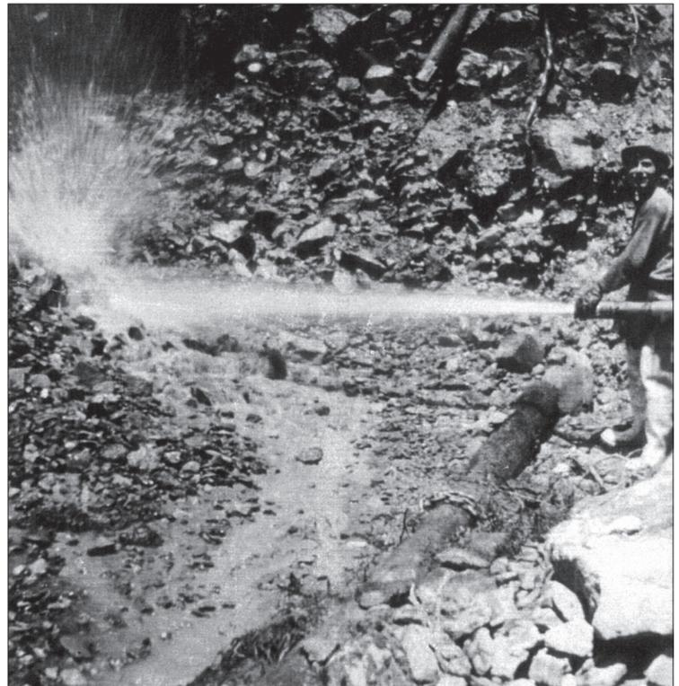
Figure 1.8. Sonny Werning mining sapphires with a hydraulic in 1937. Judging from the date and the thickness of the gravel, this may have been Coal Gulch. Photo provided by Chris Cooney.
